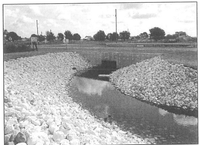
Relevancy - Earthwork and Road Crossing w/ Cast-In-Place Box Culvert
