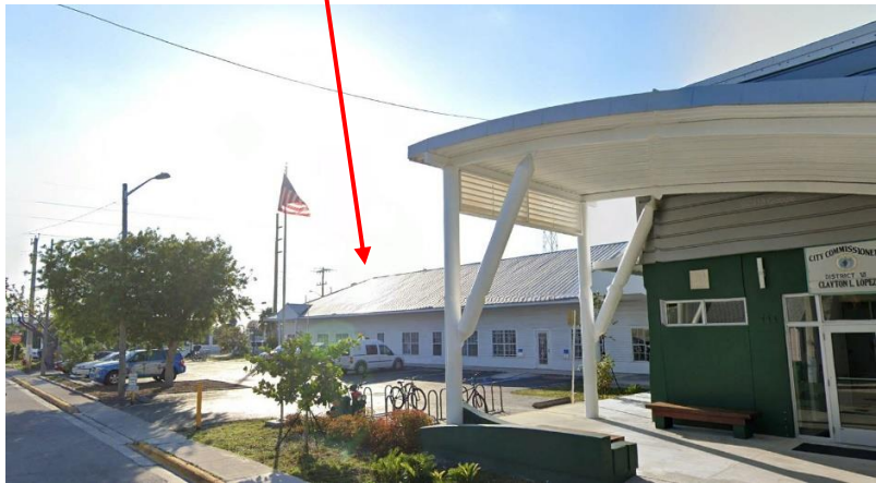
The existing Annex Building
