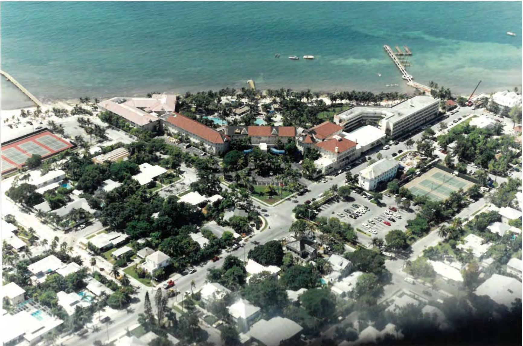
Aerial photograph of Casa Marina September 1, 1999. City of Key West.
