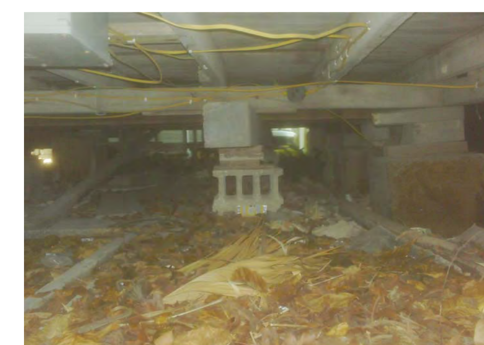
EXISTING CRAWLSPACE PIER CONDITION
