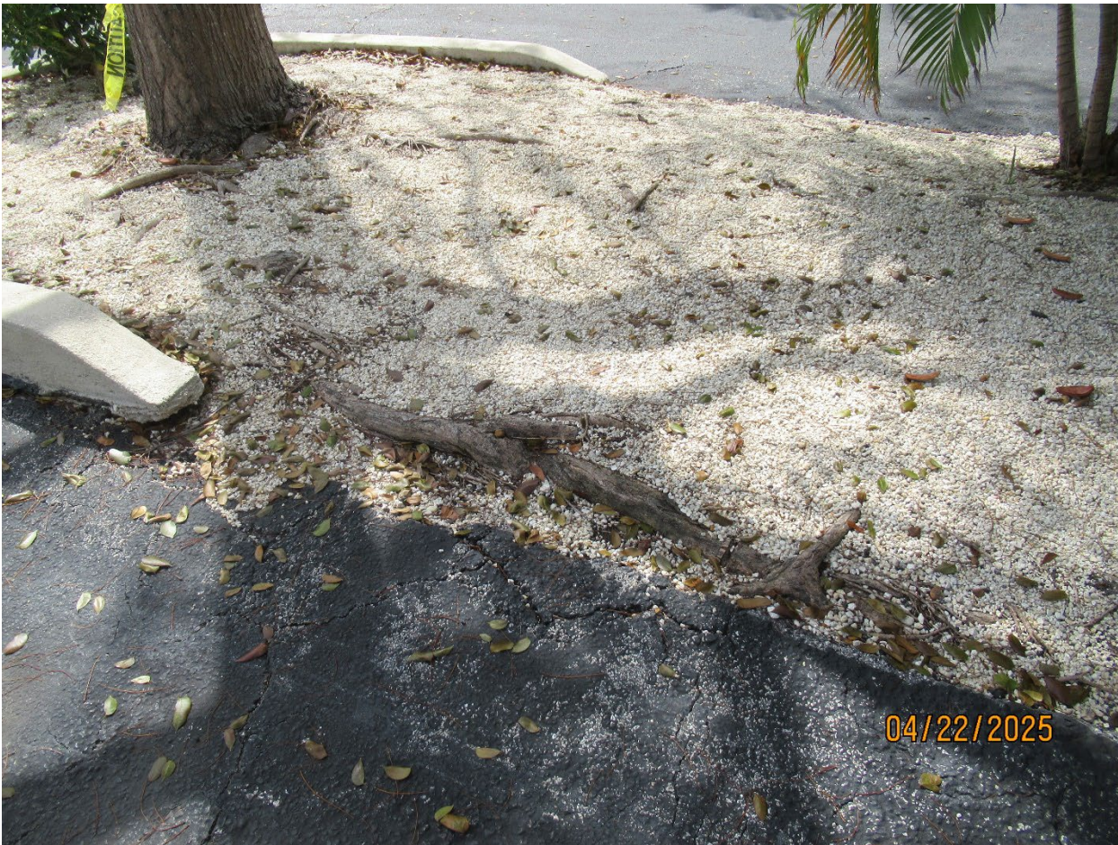
A photo of the tree's roots lifting and cracking the driveway
