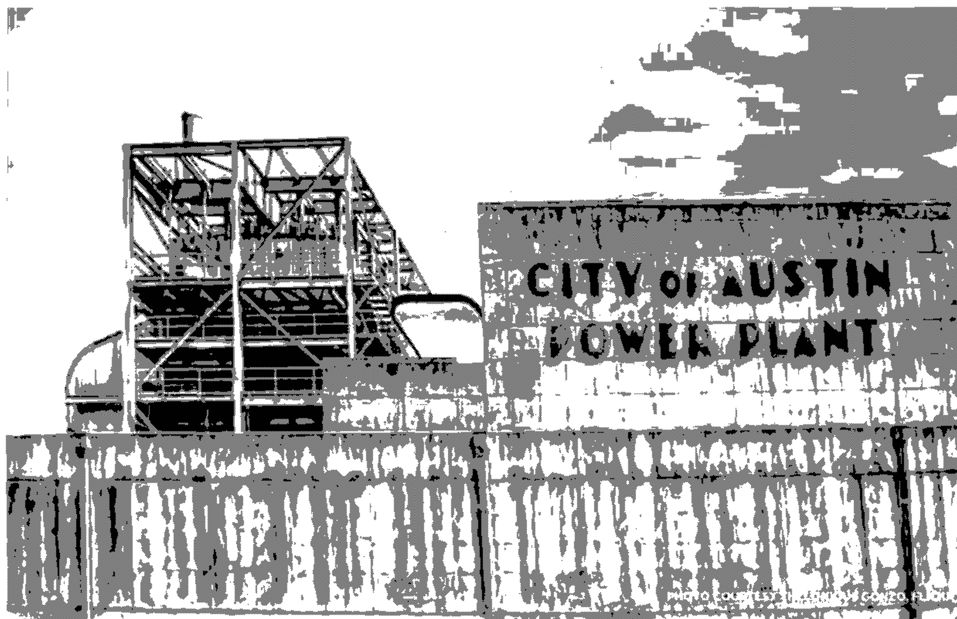
Seaholm Power Plant in Austin, Texas.
