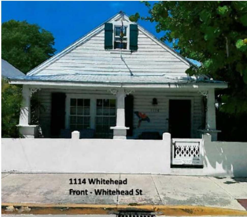
Current photo of house under review.
