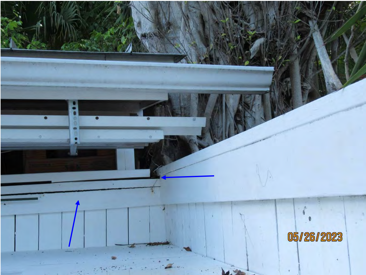
Photo showing location of neighboring structure and tree. Note impact area on structure.
