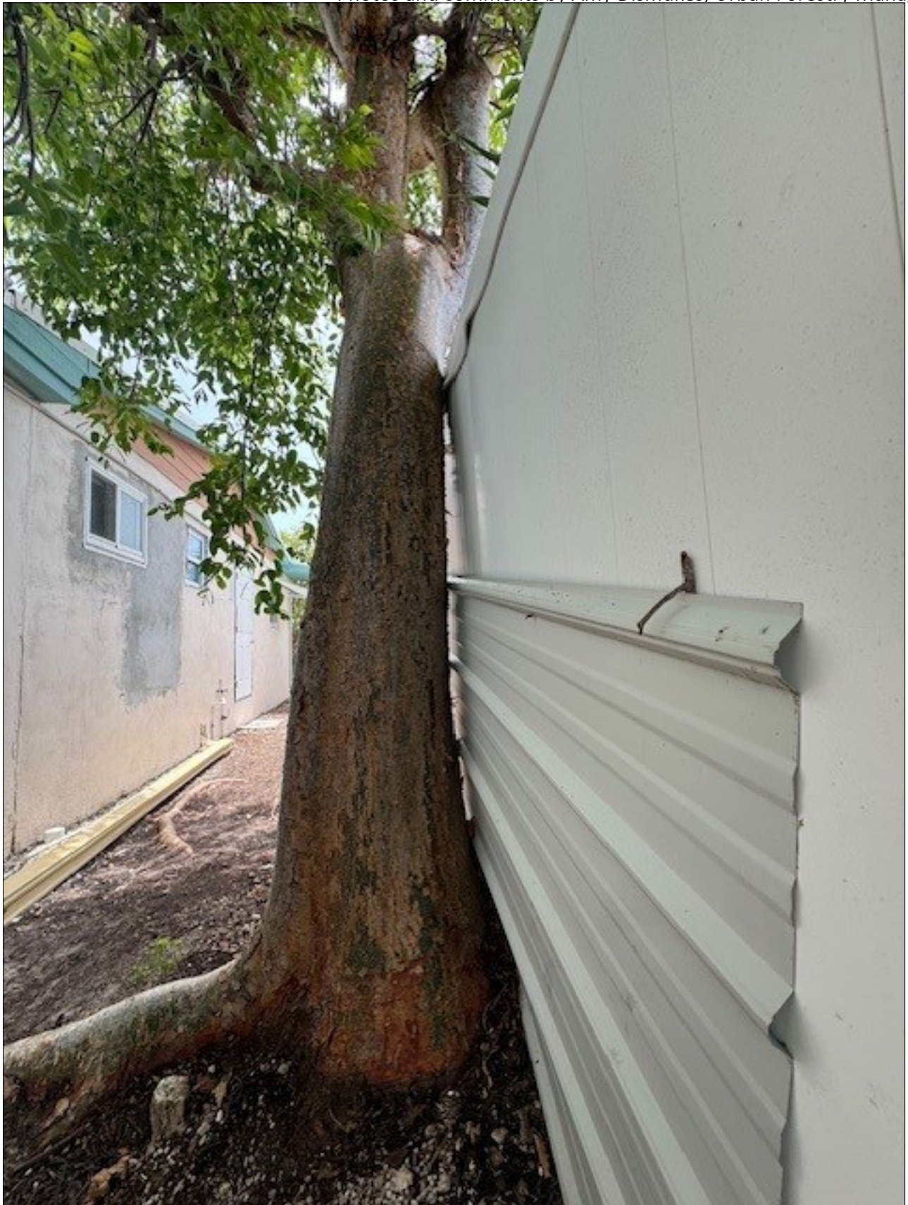
View of the tree from the canal, growing against and under the wall.
