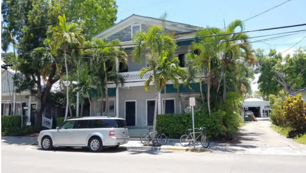
Adjacent building, 320 Simonton.
