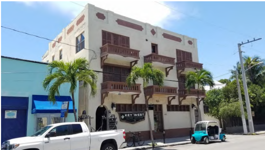
Adjacent building, 314 Simonton
