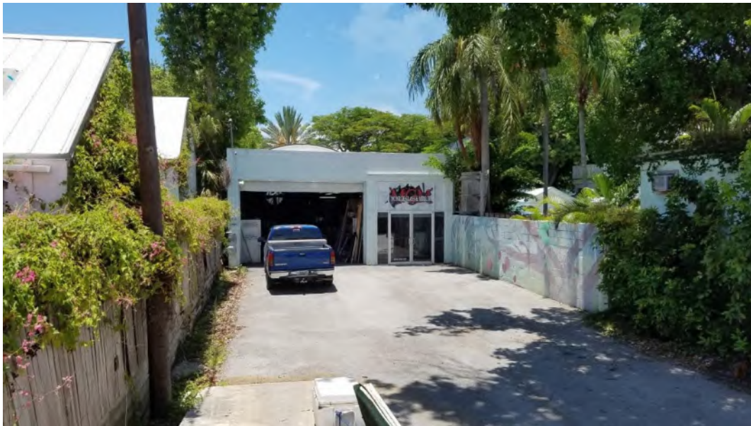
Building 5, the existing building at rear of site. Remove garage door and install storefront glass to convert to office space.
