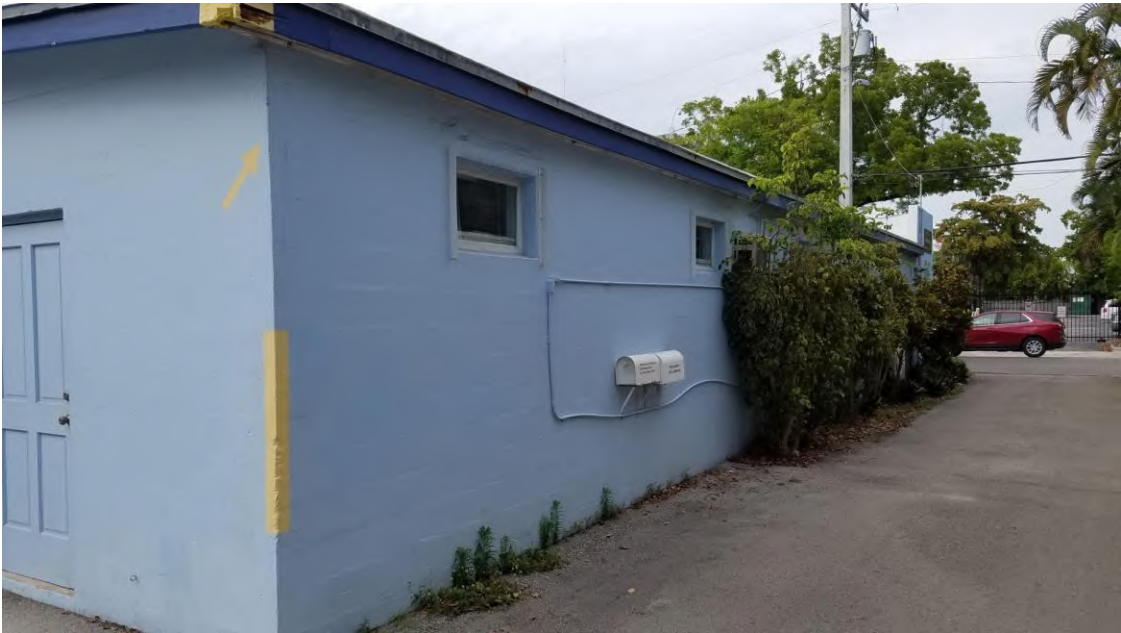
South side of building 2.
