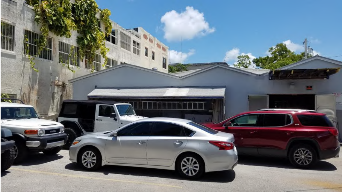
Building 3 Exterior, east side
