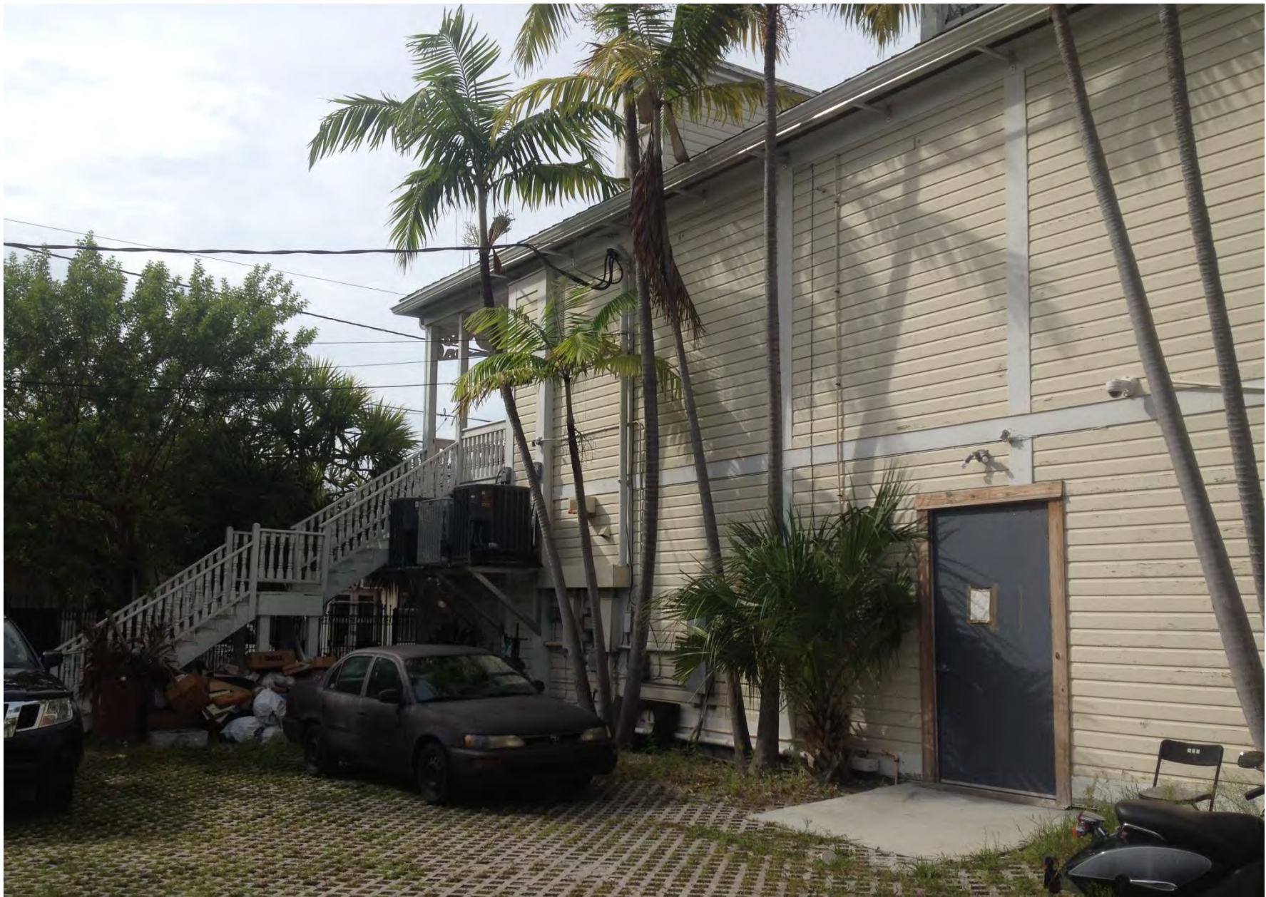
725 Duval Street PARTIAL REAR VIEW
