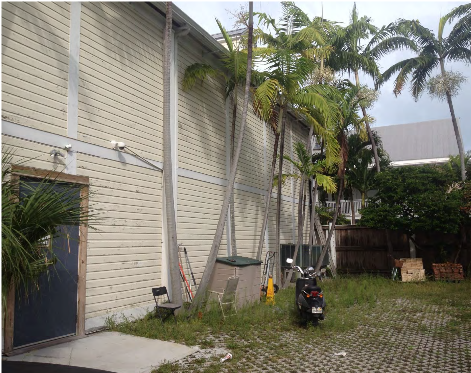
725 Duval Street PARTIAL REAR VIEW
