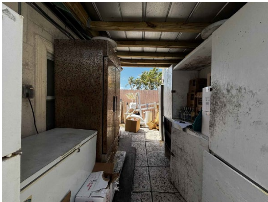
Existing Accessory Structure (South Elevation)
