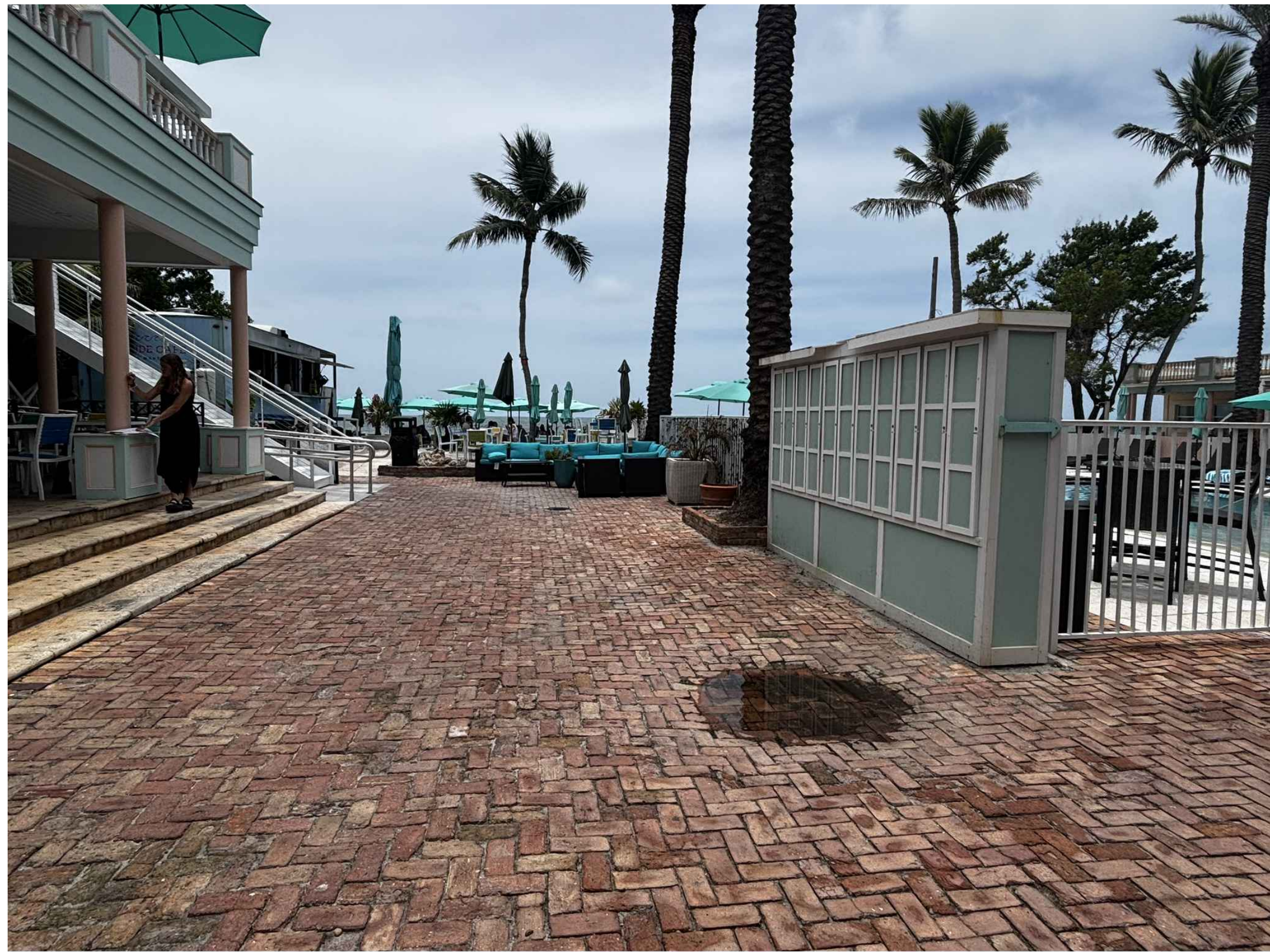
1 A6 PHOTOGRAPH OF AREA FOR NEW BATHROOMS (SOUTH VIEW) SCALE: N.T.S.
