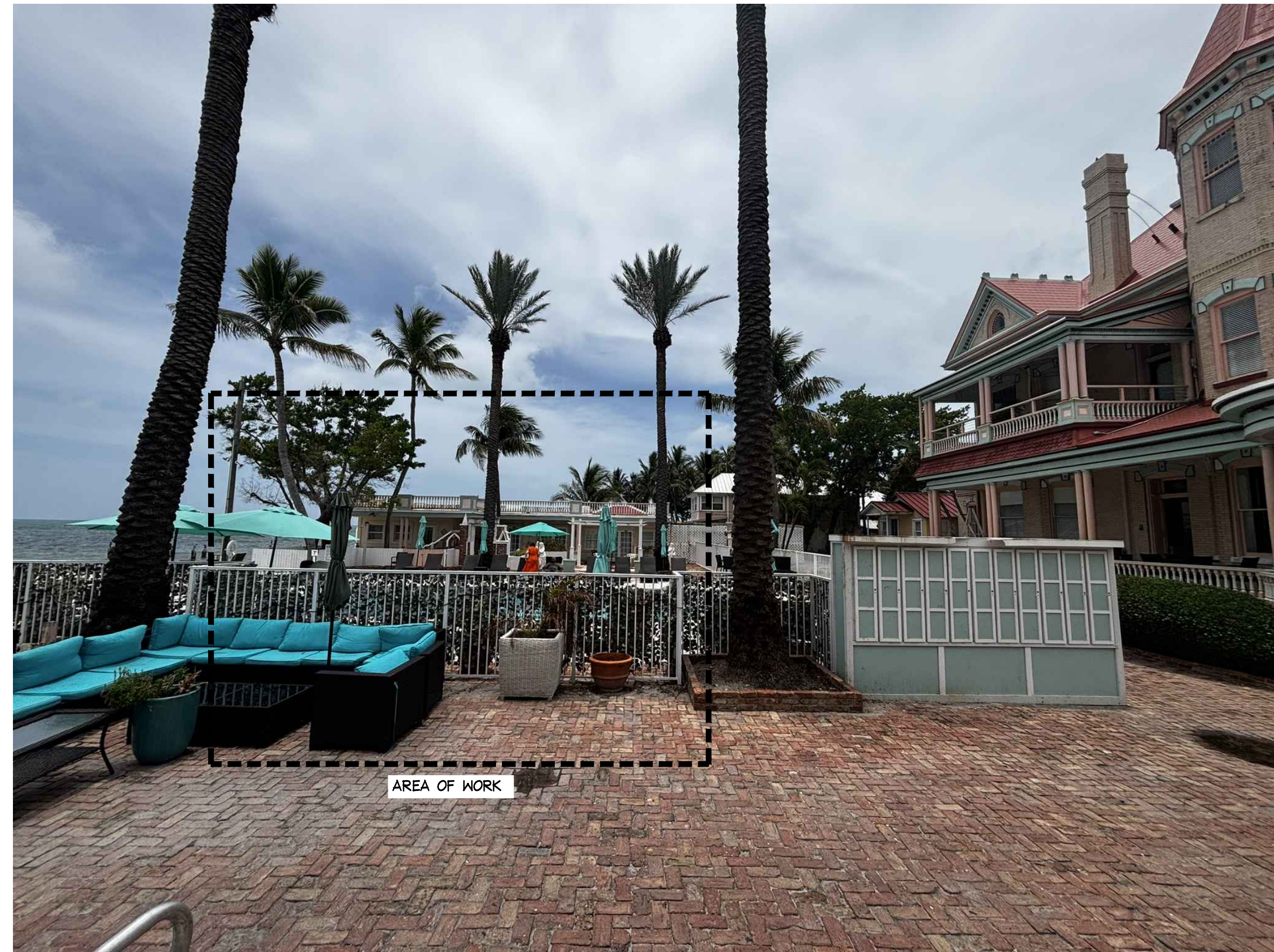
1 A6 PHOTOGRAPH OF AREA FOR NEW BATHROOMS (WEST VIEW) SCALE: N.T.S.
