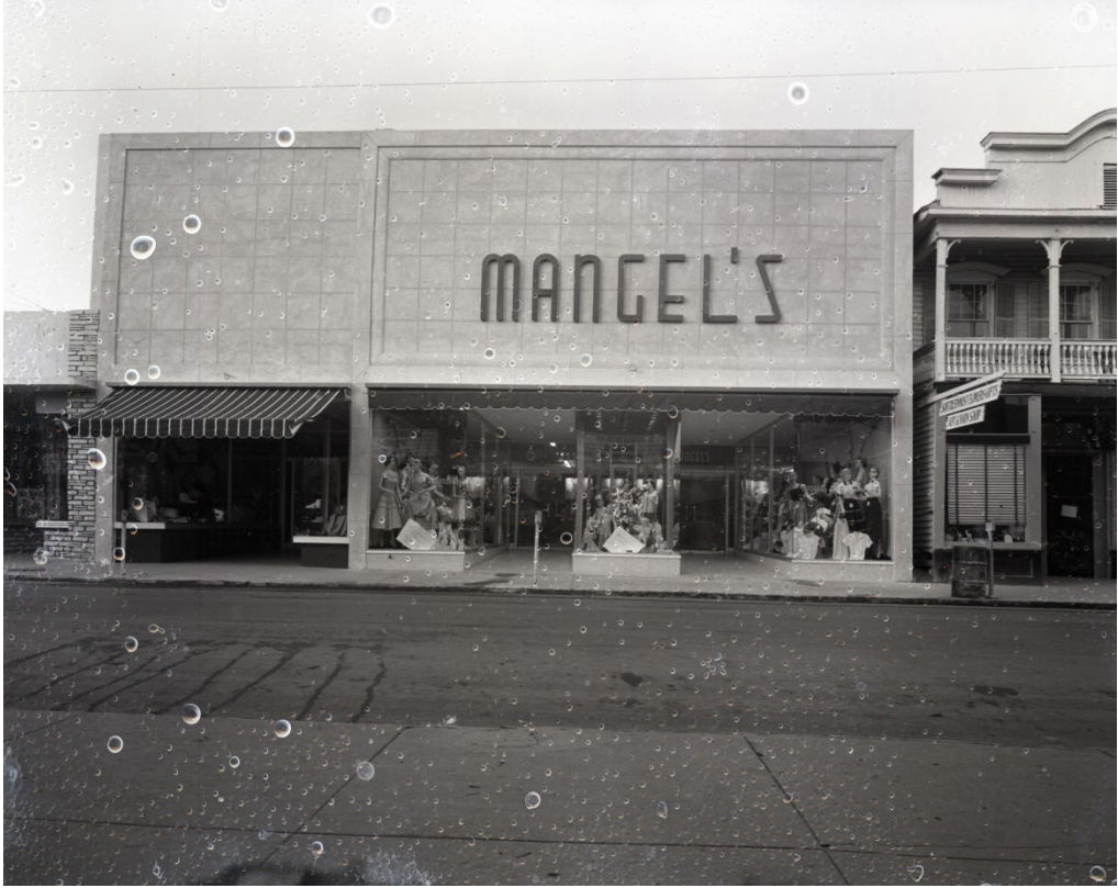
c. 1954 Historic Photo of Property Under Review.
