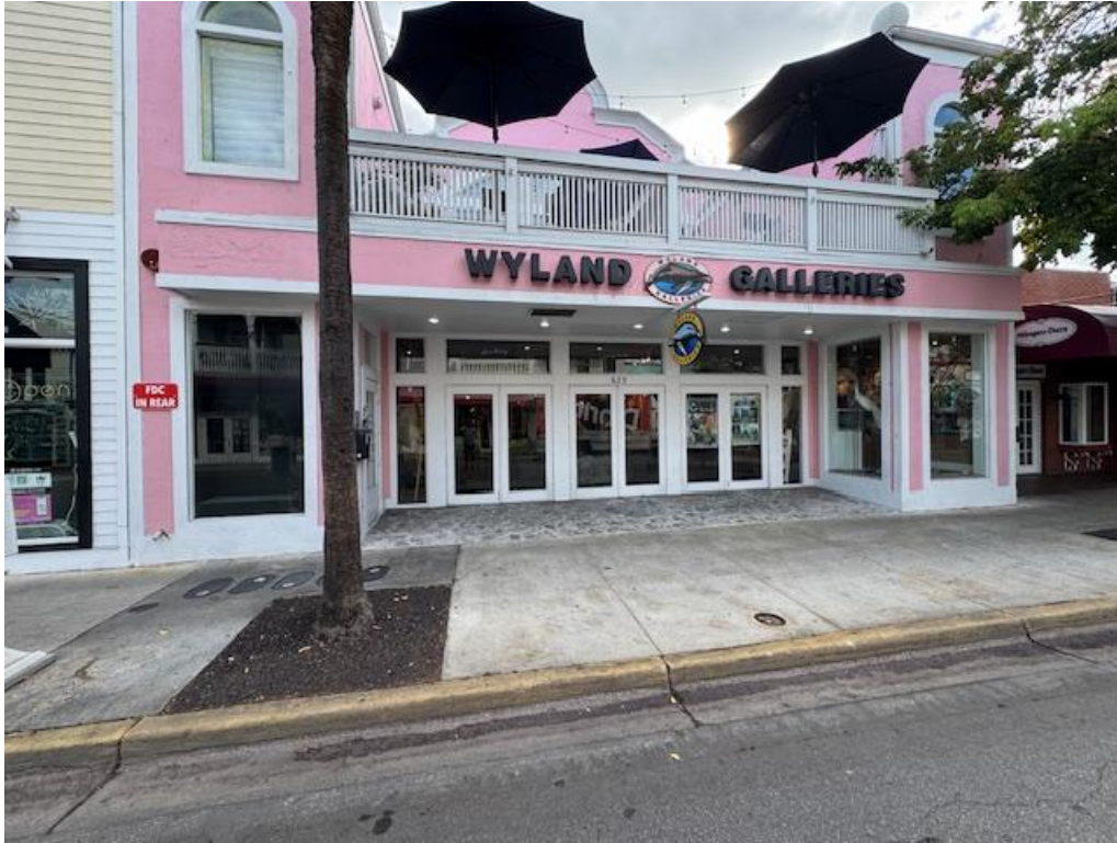
Photograph of 623 Duval structure – Wyland Galleries with folding doors.
