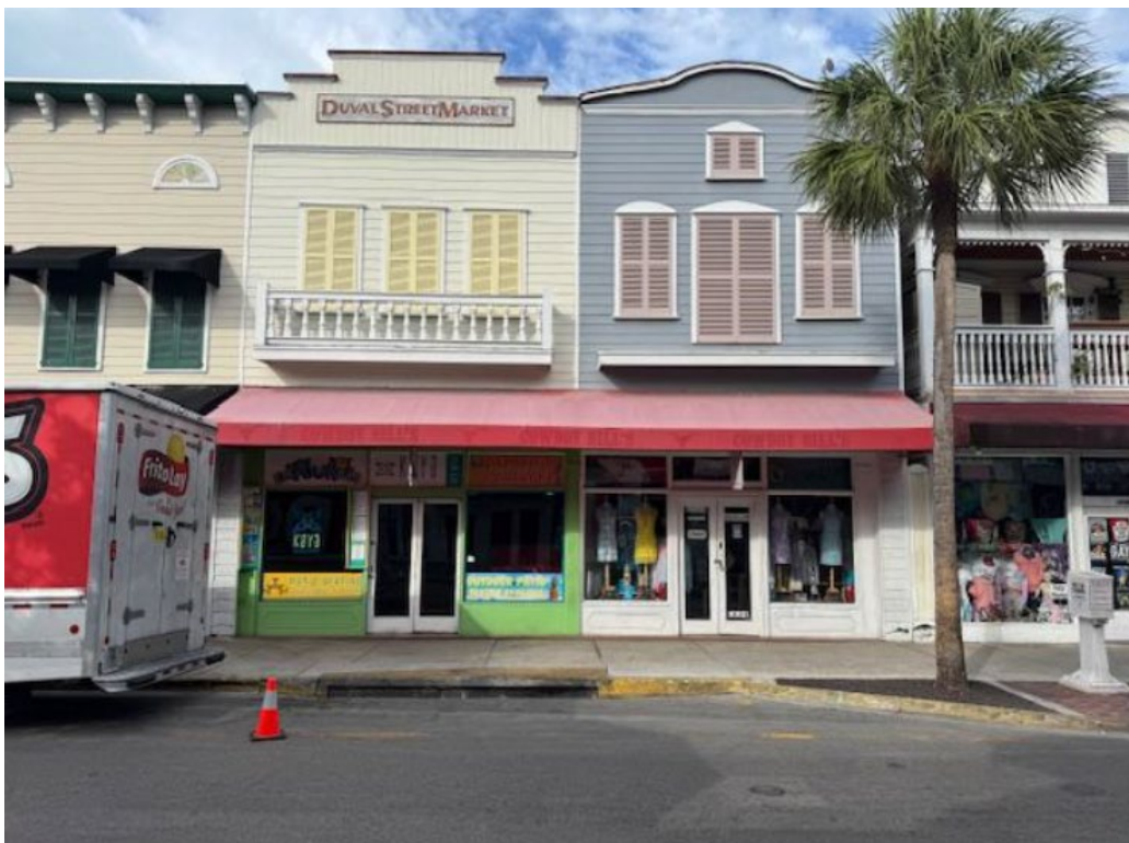
Photo of Property Under Review and Adjacent Structure.
