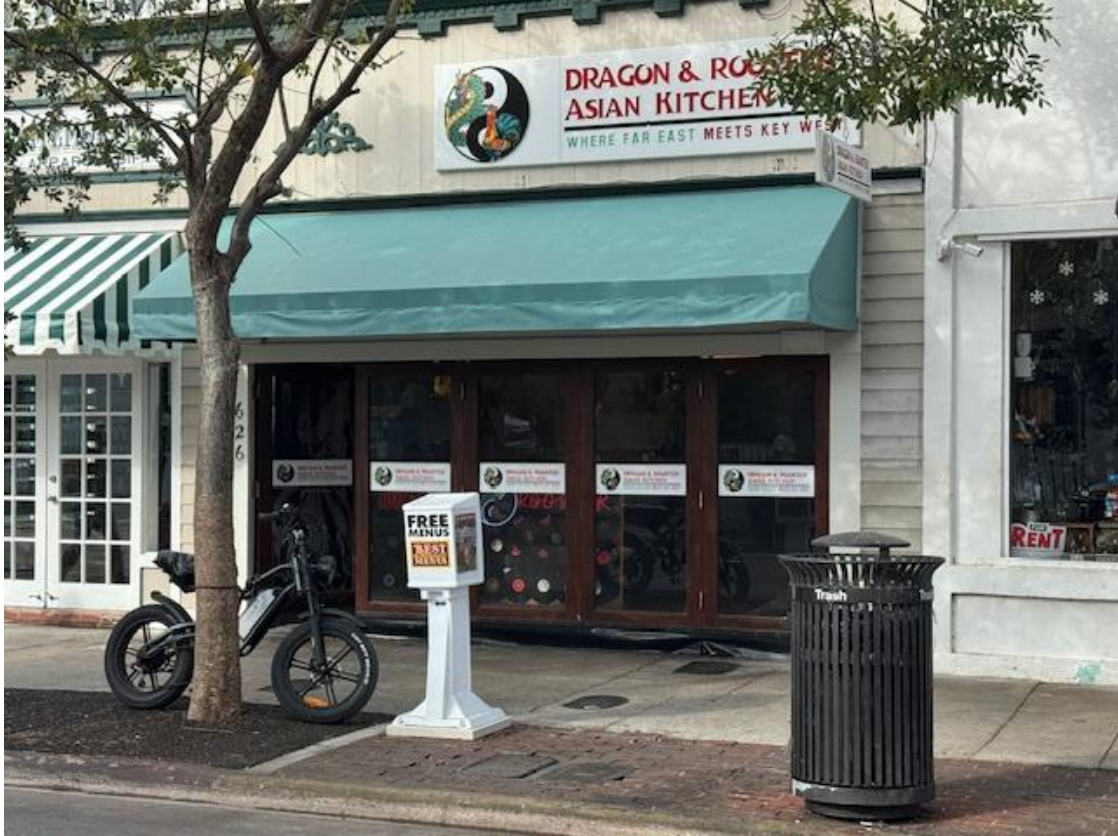
Photograph of 626 Duval structure with folding doors.
