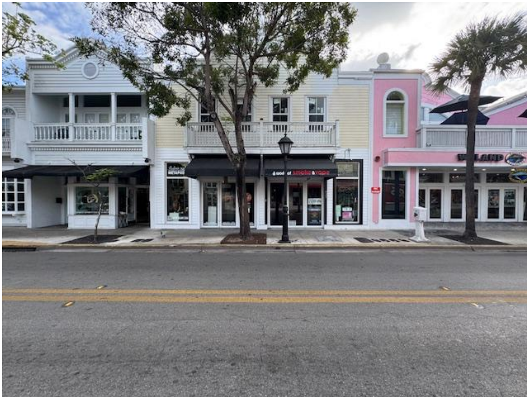
Photograph of 619 Duval structure with folding doors.
