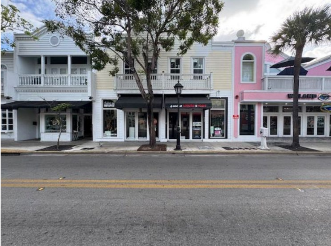
Photo of 619 Duval Street Showing Storefront Similar to Proposed Storefront for 618 Duval Street.
