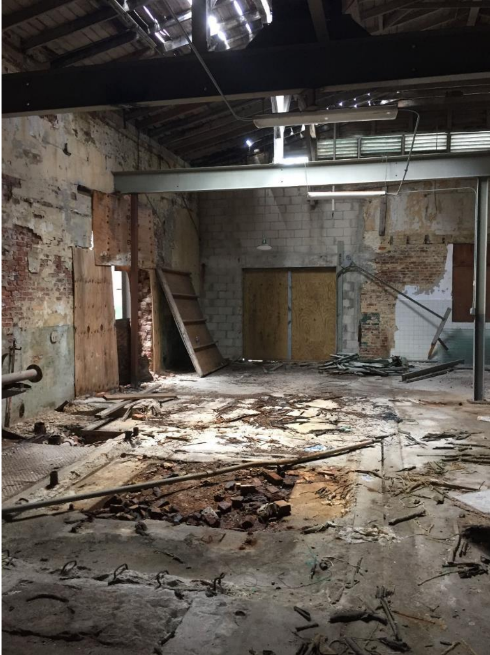
PHOTO 4: Interior of buildings at the Site
