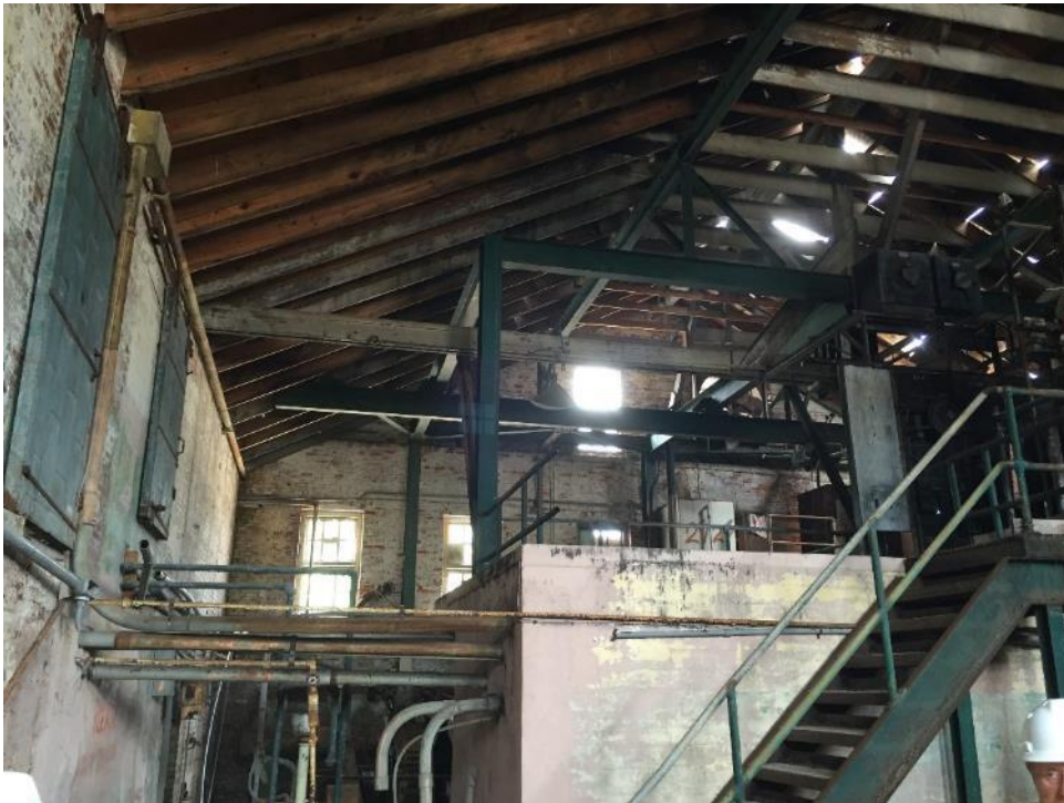
PHOTO 10: Interior of buildings at the Site
