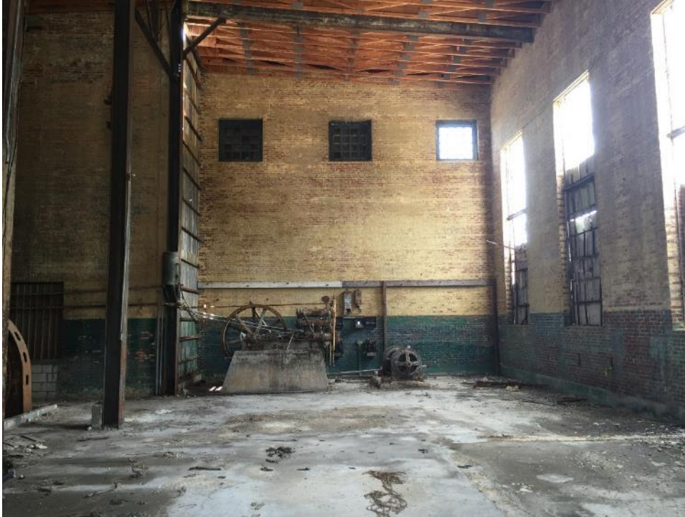
PHOTO 5: Interior of buildings at the Site
