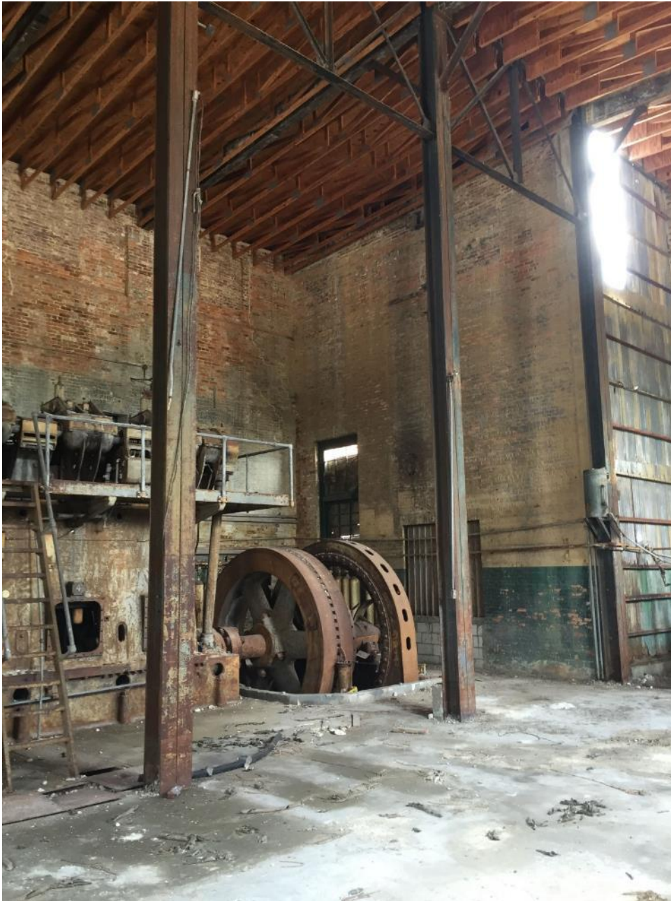
PHOTO 6: Interior of buildings at the Site showing an inactive generator
