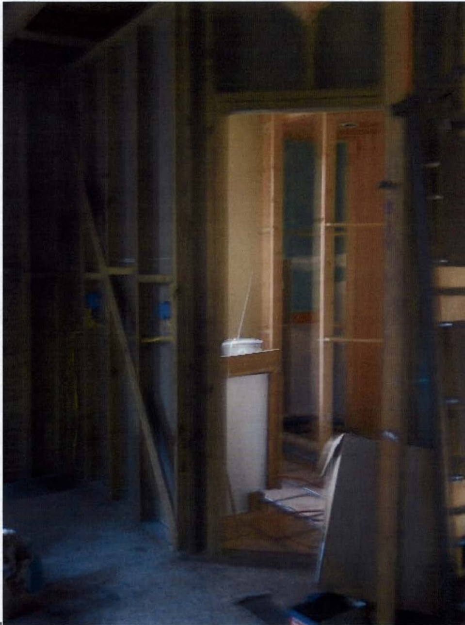
I found some Dade county pine in the "attic". I cleaned it up, scraping and sanding and used it on the knee walls of the shower...
