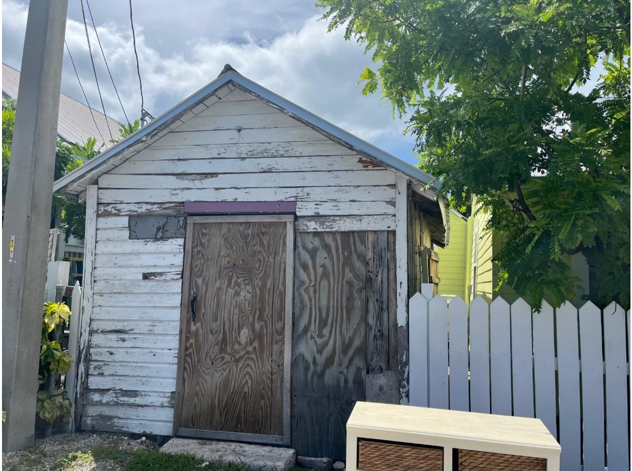
Photo 2 of the front of the historic accessory structure at 205 Julia Street.
