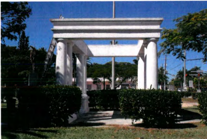
View of South Elevation of Civil War Memorial
