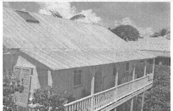
Overview roof - right side- Standing seam metal
