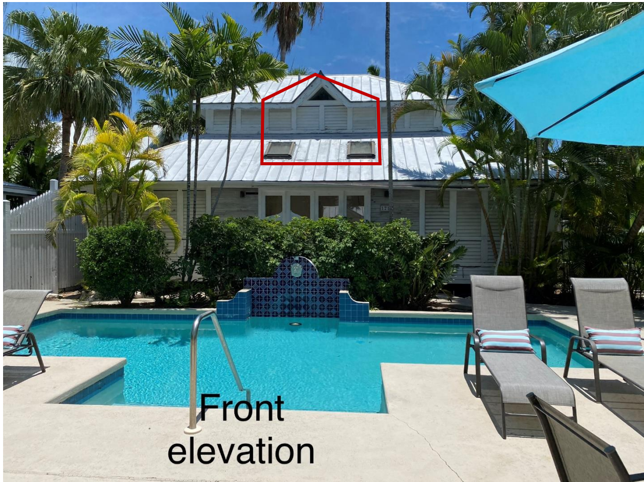
Photograph of the house front elevation with proposed demolition marked in red.
