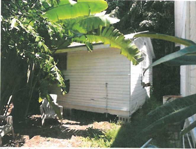
View of the west side of the secondary structure
