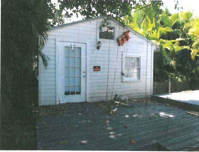
View of the front of the secondary structure behind the main structure
