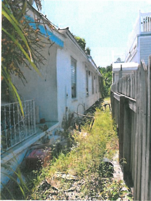
View of west side of main structure
