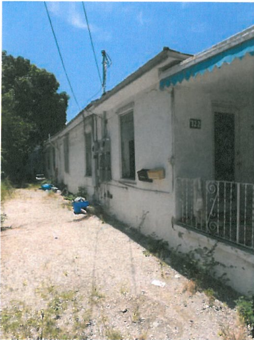
View of east side of main structure
