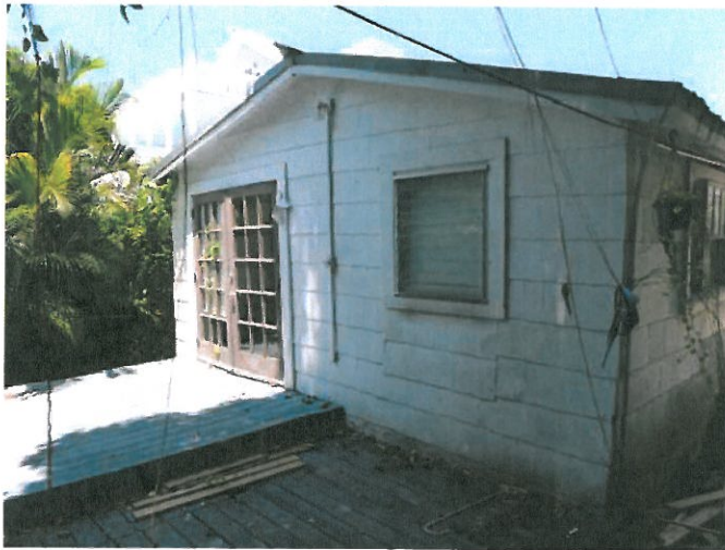
View of the rear of the main structure
