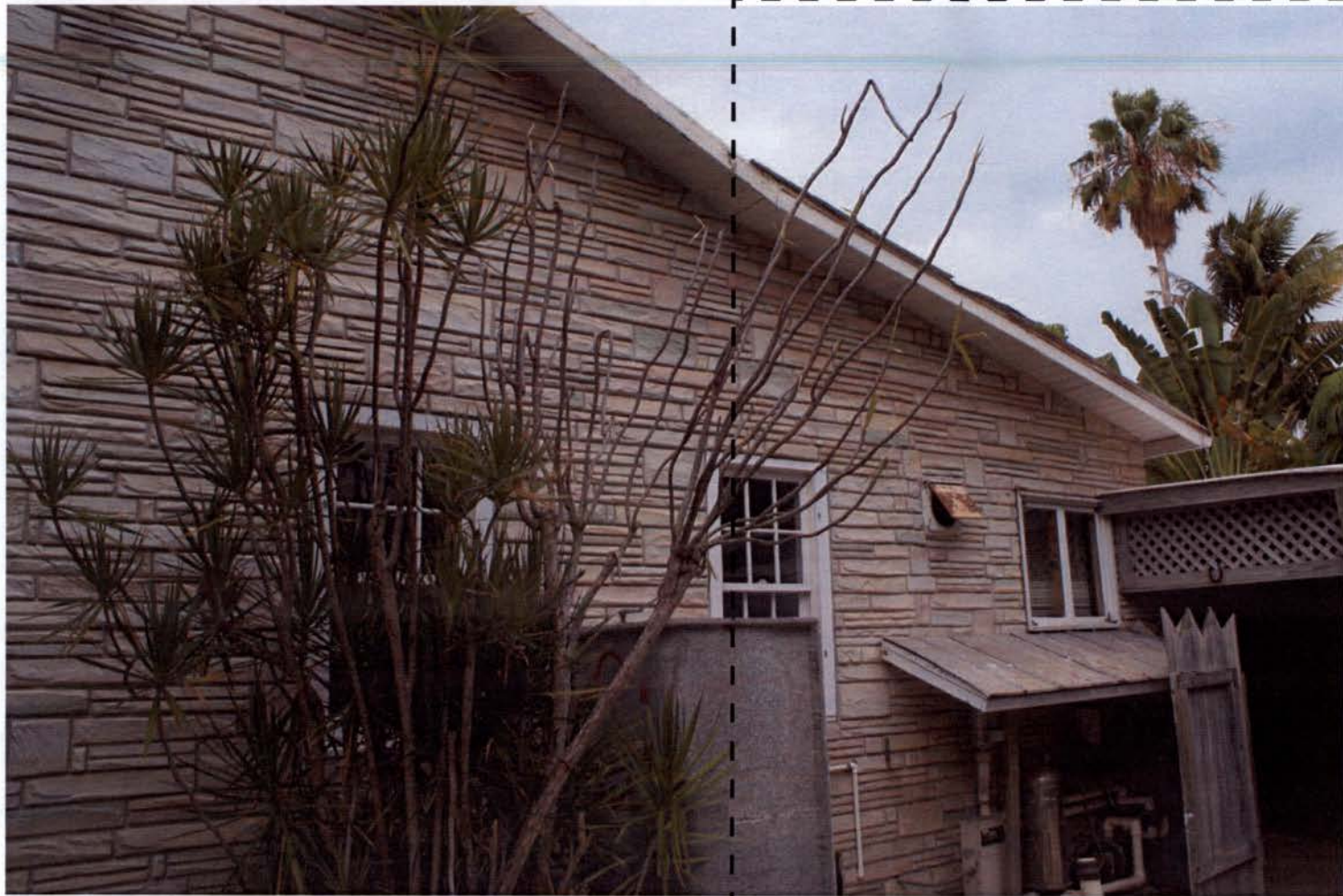
Photograph looking at West facade of existing building
