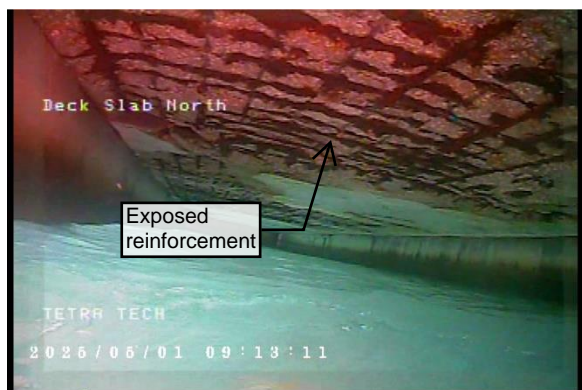
Figure 3 – Exposed reinforcing steel on underside of deck slab
