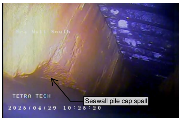
Figure 34 – Spalling on bottom face of sheet pile cap
