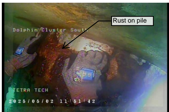
Figure 55 – Rust on pile of south dolphin
