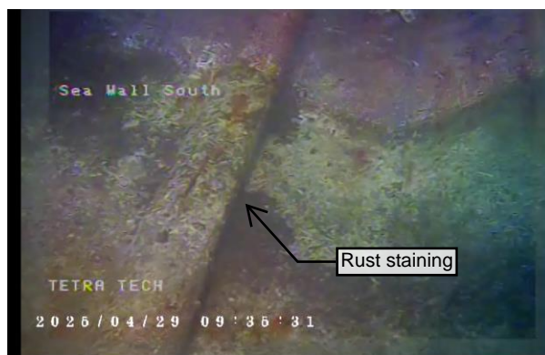
Figure 31 – Typical photo of sheet pile under water line
