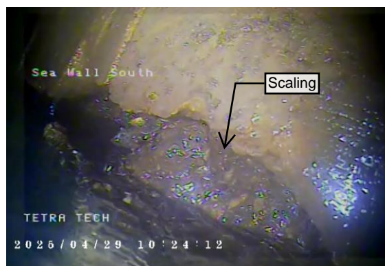
Figure 35 – Scaling on bottom face of sheet pile cap
