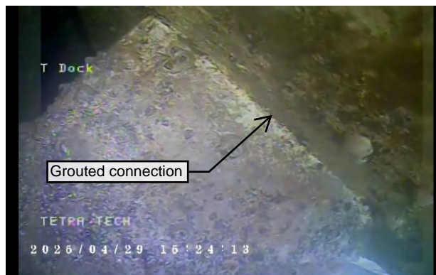
Figure 45 – Pile to pile cap connection
