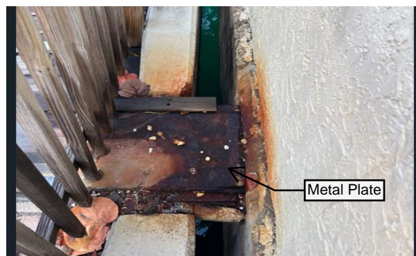
Figure 24 – Metal plate with rust stains.
