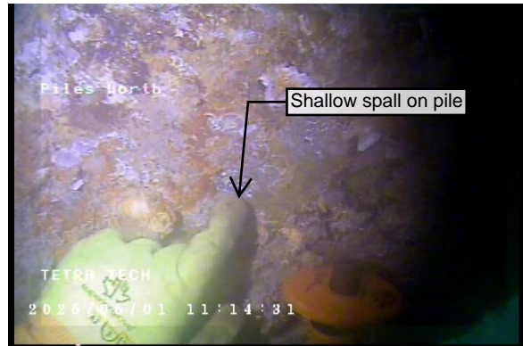
Figure 12 – Minor spall on pile cap
