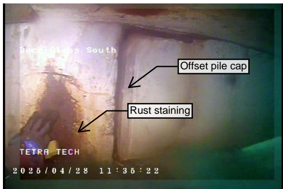
Figure 21 – Rust and separation on joint
