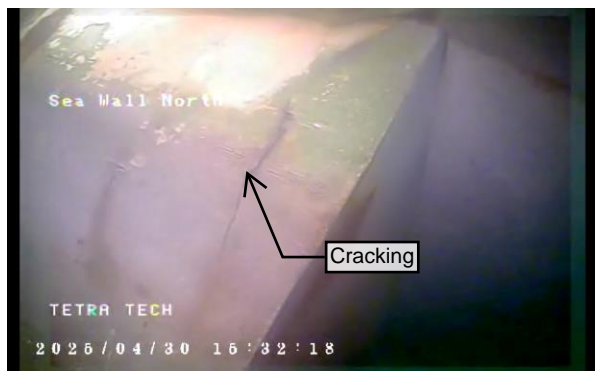
Figure 23 – Diagonal crack on Bent C
