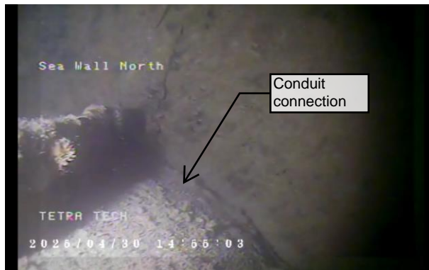
Figure 39 – Top of conduit connection
