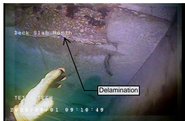
Figure 8 – Delamination on underside
