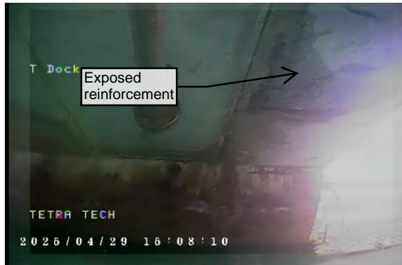
Figure 42 – Exposed reinforced steel on decking
