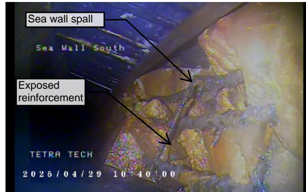
Figure 38 – Exposed reinforcing steel on sheet pile cap
