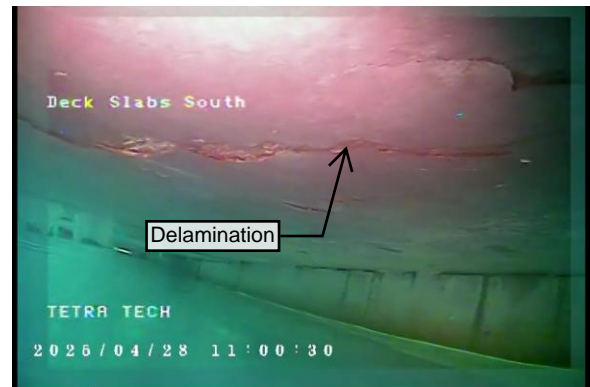
Figure 6 – Delamination on underside decking
