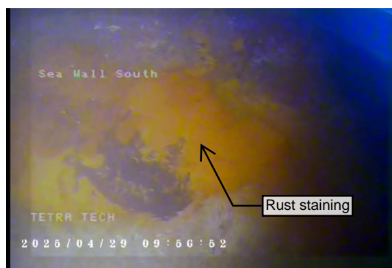
Figure 33 – Rust staining under water line
