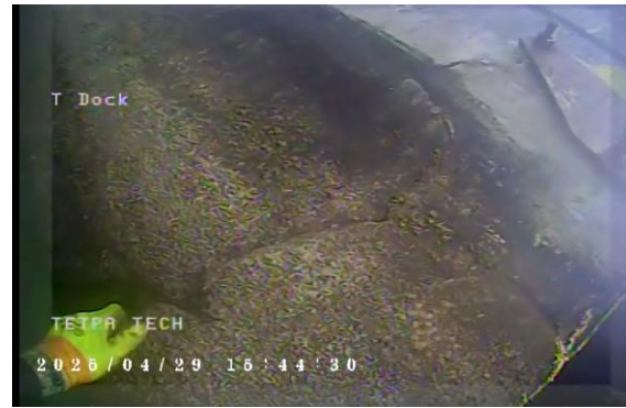
Figure 52 – Crack on corner of south T-dock dolphin
