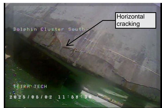
Figure 56 – Cracking on face of south dolphin
