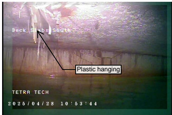
Figure 5 – Hanging plastic on underside decking
