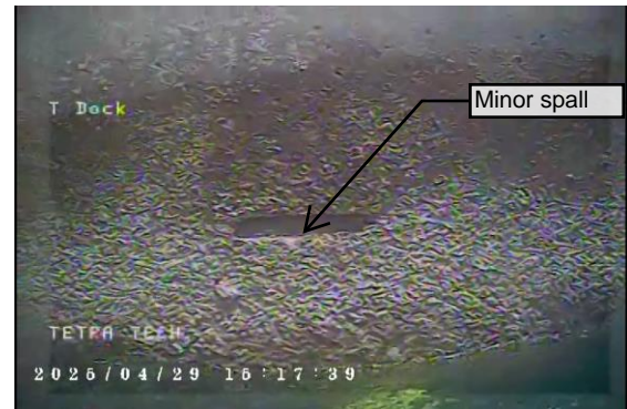
Figure 54 – Minor spall and scaling on pile cap
