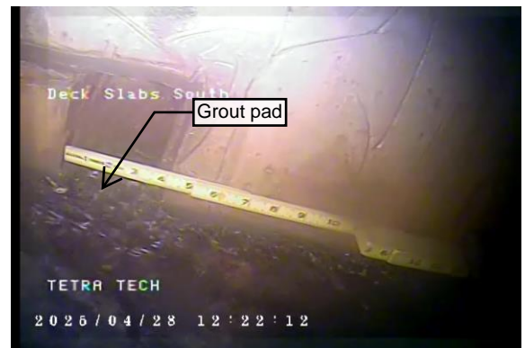
Figure 22 – Degradation of 1/2" grout pad on Bent B
