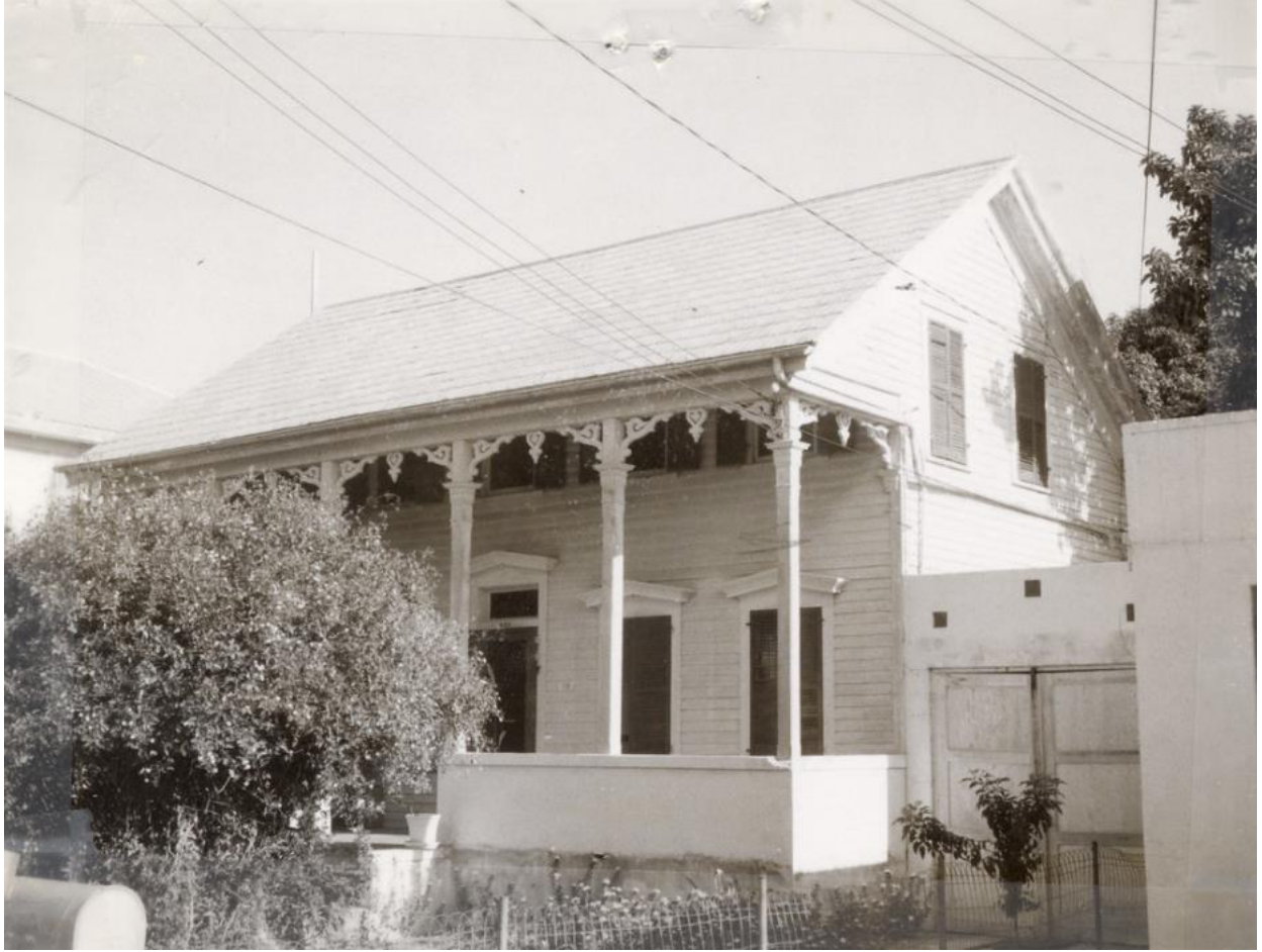
1965 photo of the house at 643 William Street.
