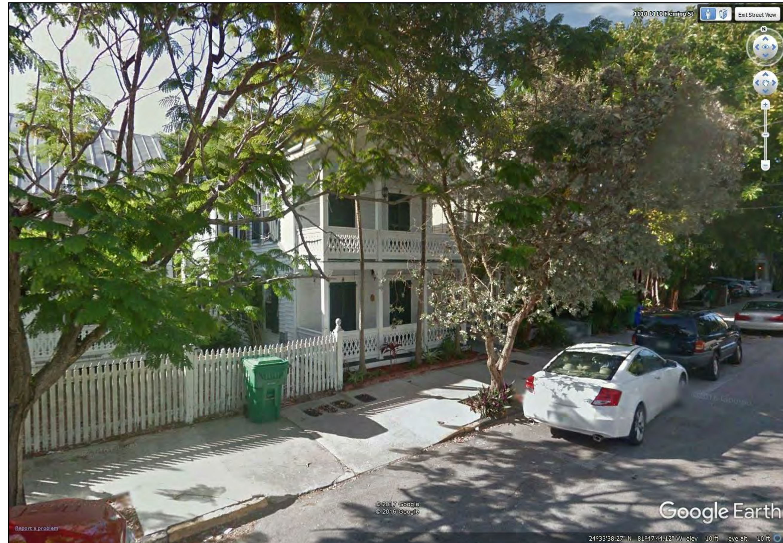
2 ADJACENT PROPERTY TO THE EAST
