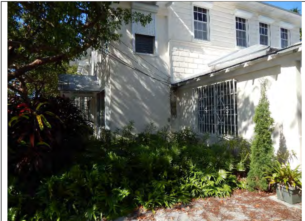
3. 1019 Flagler. View from east driveway.
