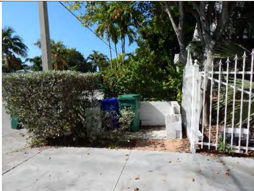
6. 1019 Flagler. Trash enclosure at west driveway.
