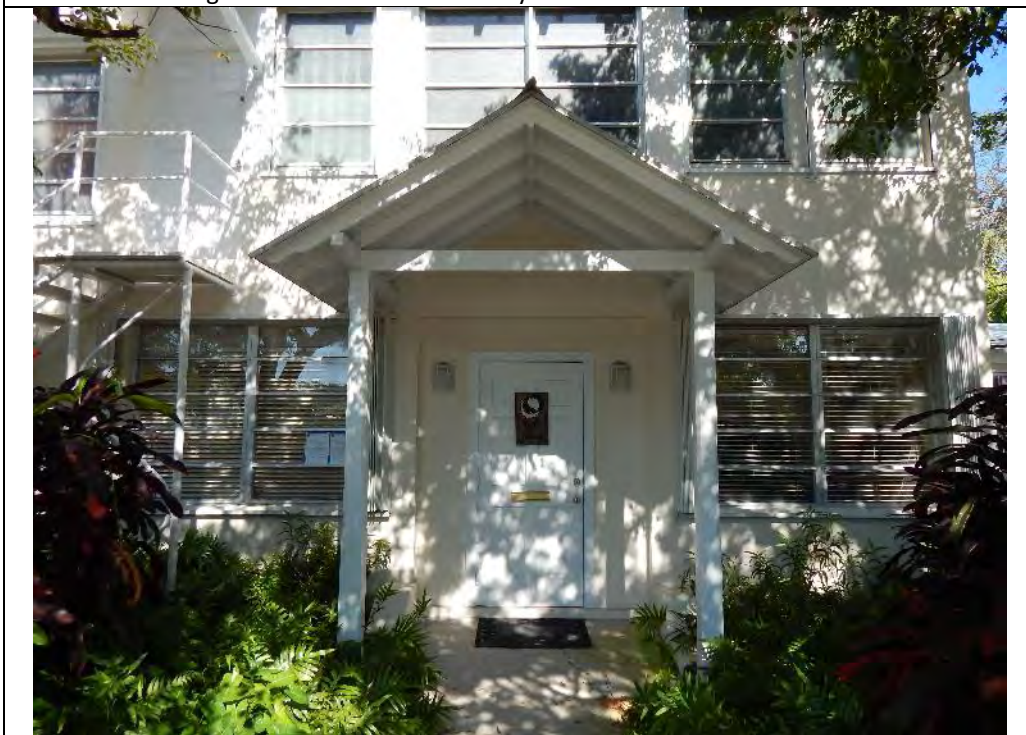
4. 1019 Flagler. Existing front addition entrance.
