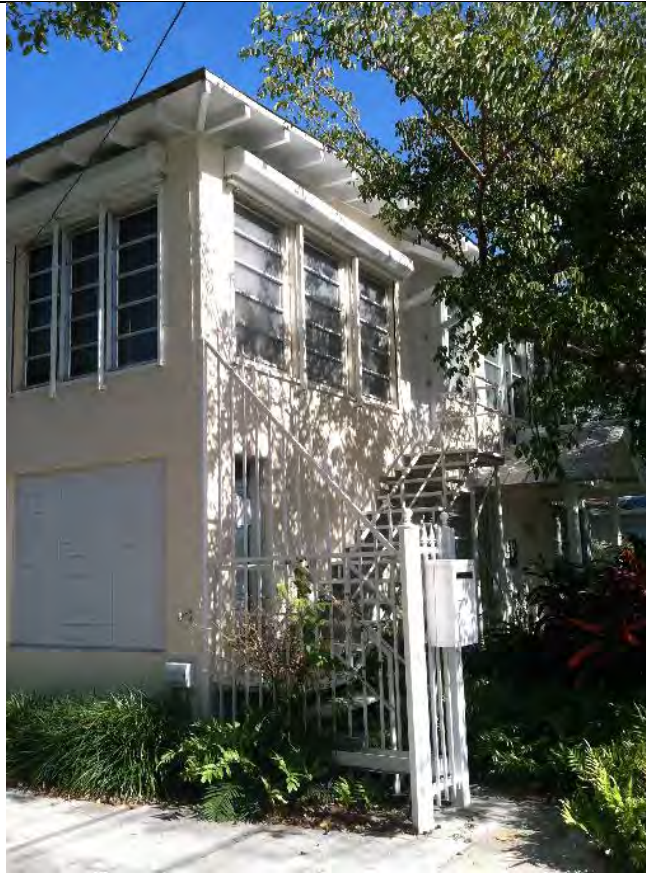
5. 1019 Flagler. View from carport / west driveway.
