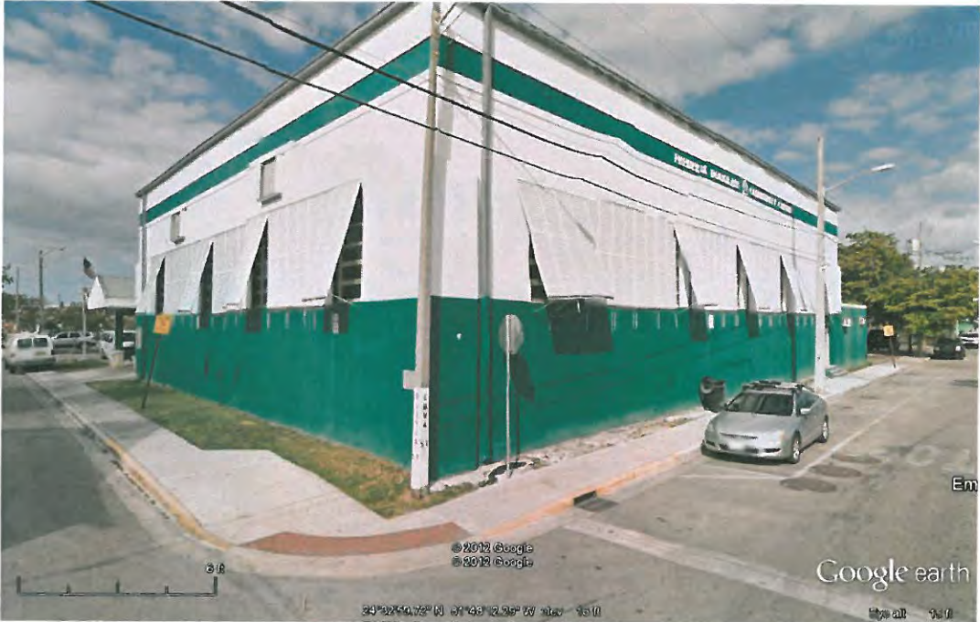
Northeast View of Building
