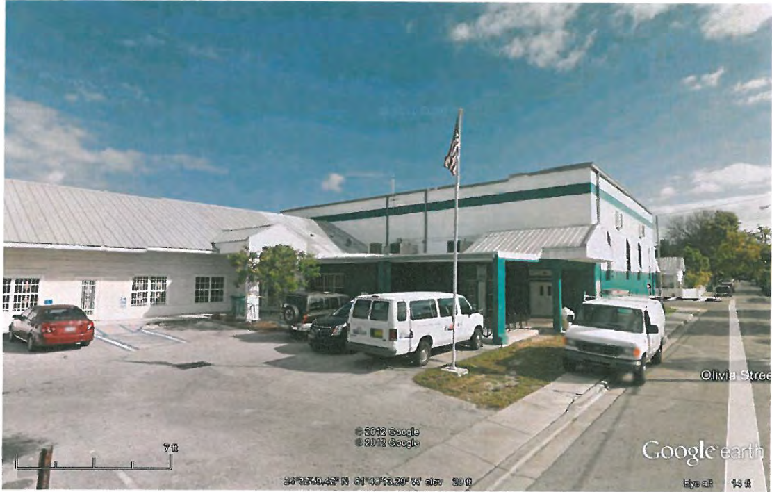
Southwest View of Building
