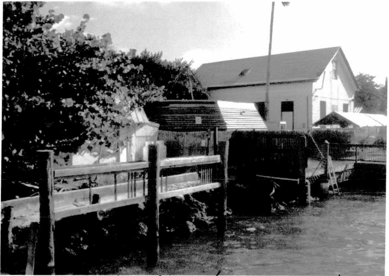
EXISTING BROKEN/ROTTED DECK BEHIND CISTERN
