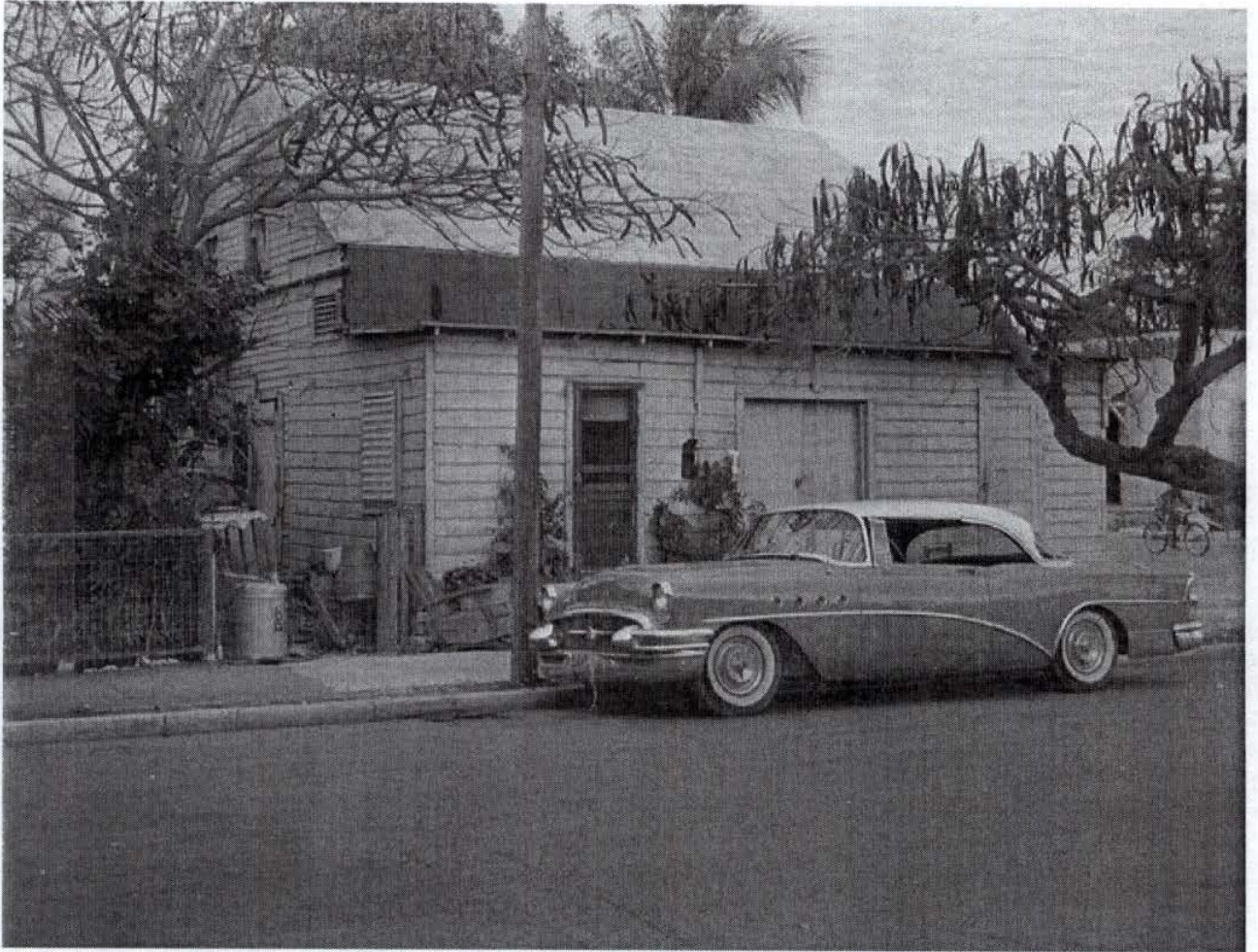
Photo taken by the Property Appraiser's office c1965; 1025 Whitehead St.; built c1892; Monroe County Library
