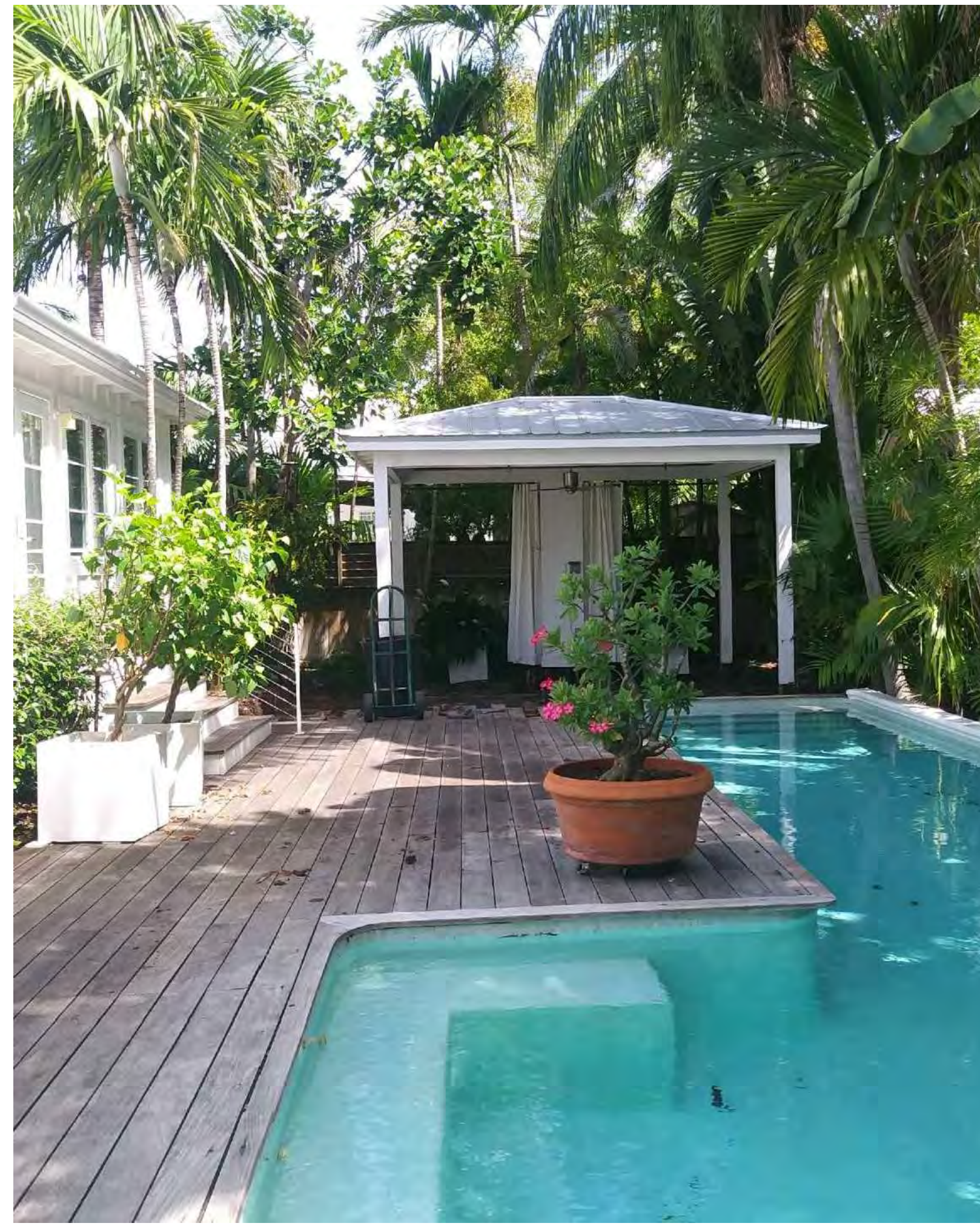
WEST ELEVATION OF EXISTING GAZEBO
