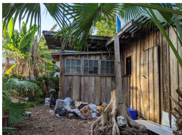
Rear view of existing structure
