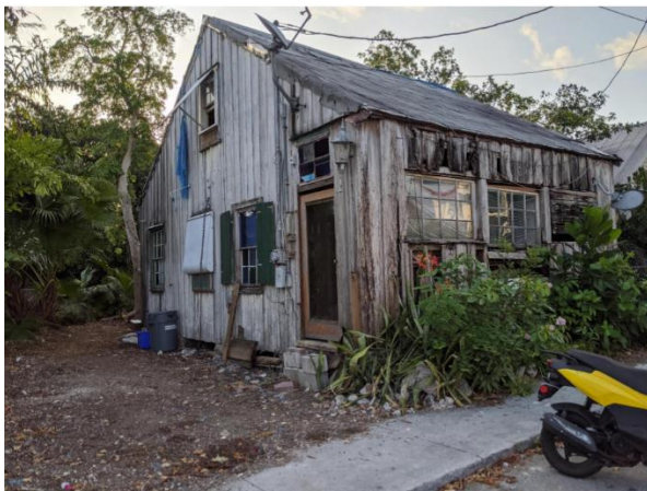
Front/side view of existing structure
