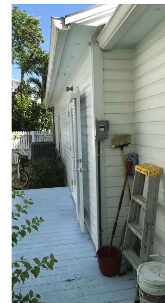
EXISTING N. SIDE OF HOUSE FROM REAR
