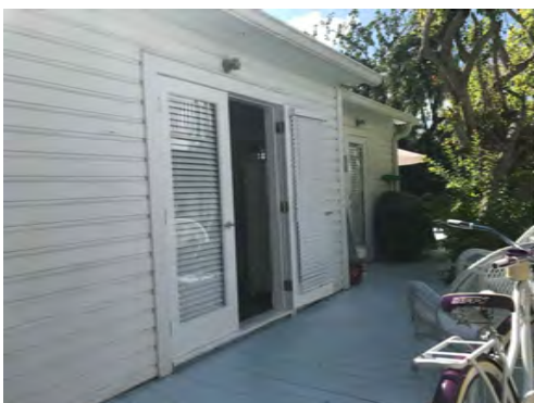
EXISTING N. SIDE OF HOUSE FROM FRONT
