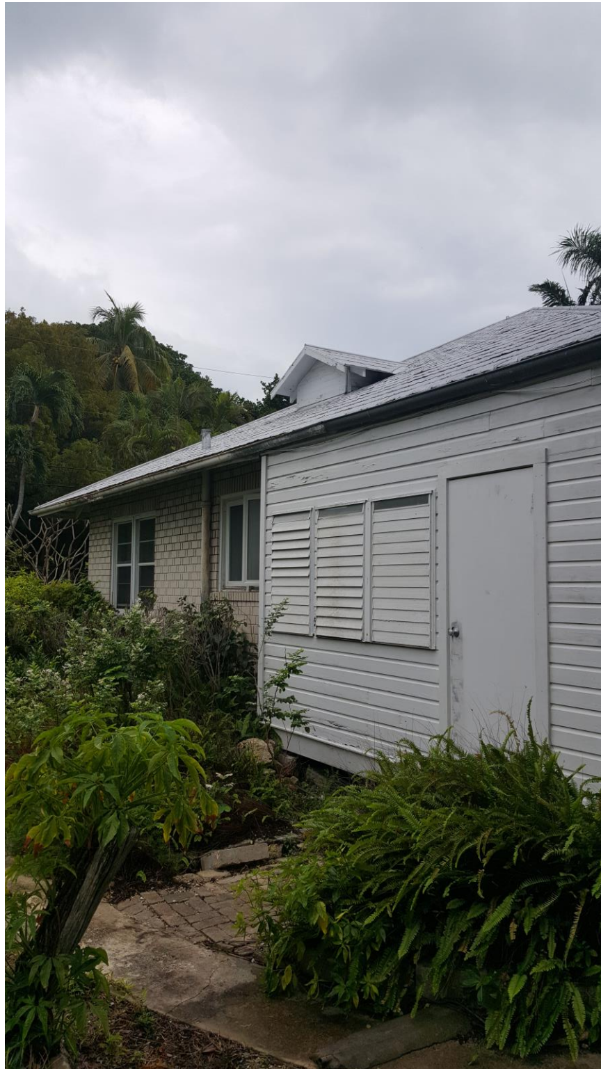
1117 South Street – Northeast Rear Addition and East Elevation
