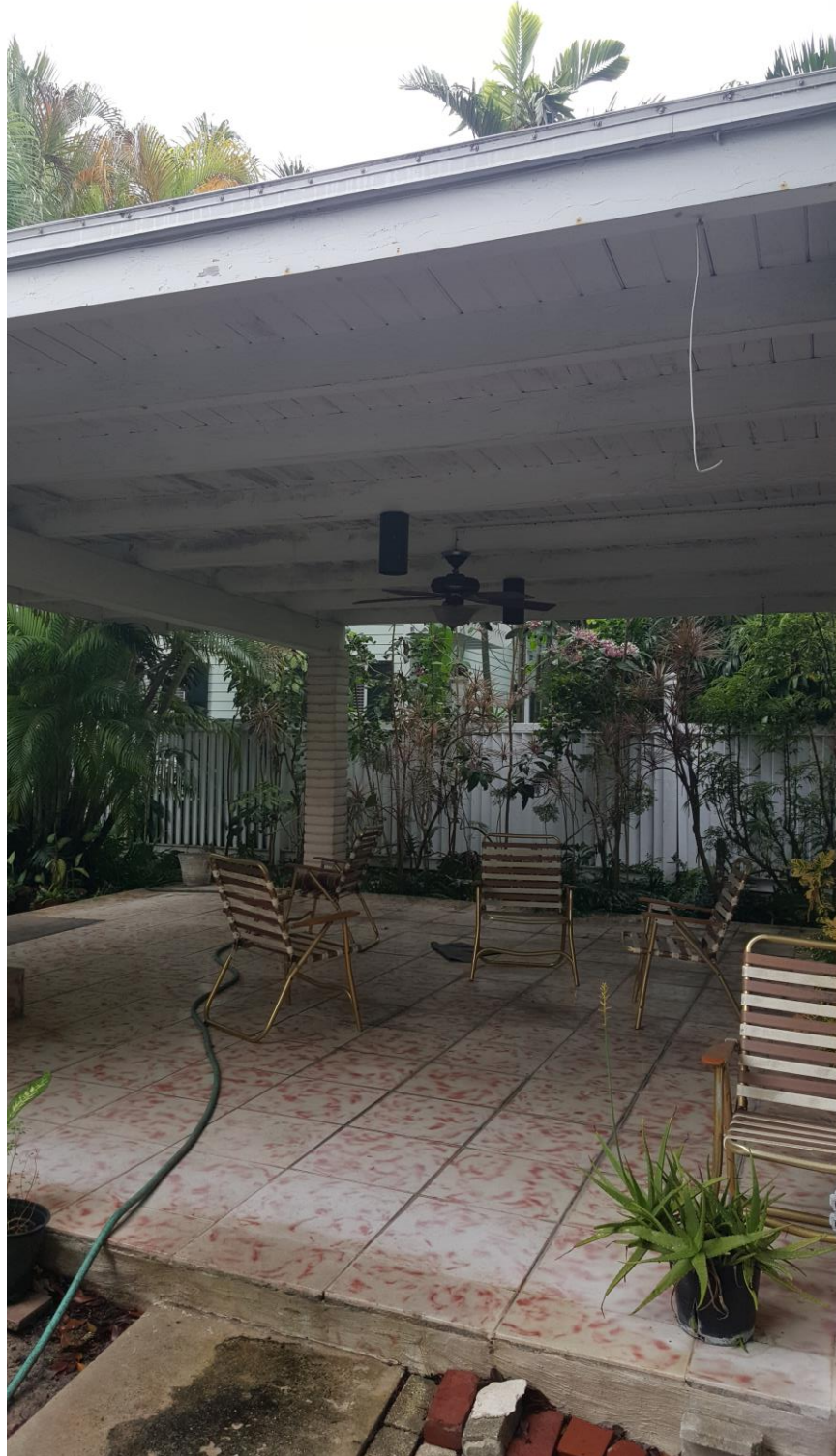
1117 South Street – Covered Patio
