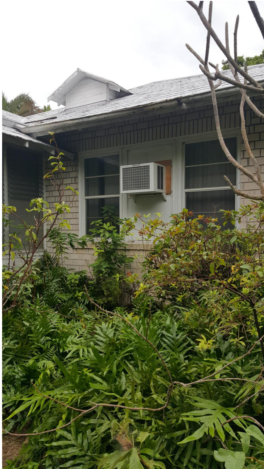
1117 South Street – Southeast Corner at Front Facade
