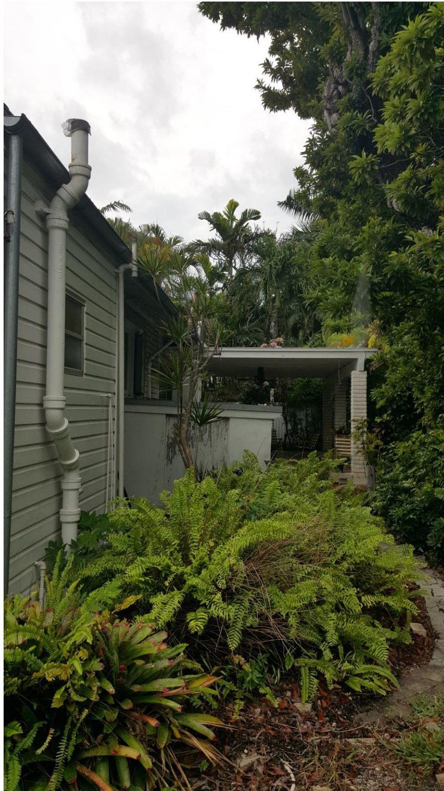
1117 South Street – Rear Additions and Covered Patio
