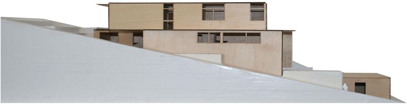
Structure Built into Base of Surrounding Slope
