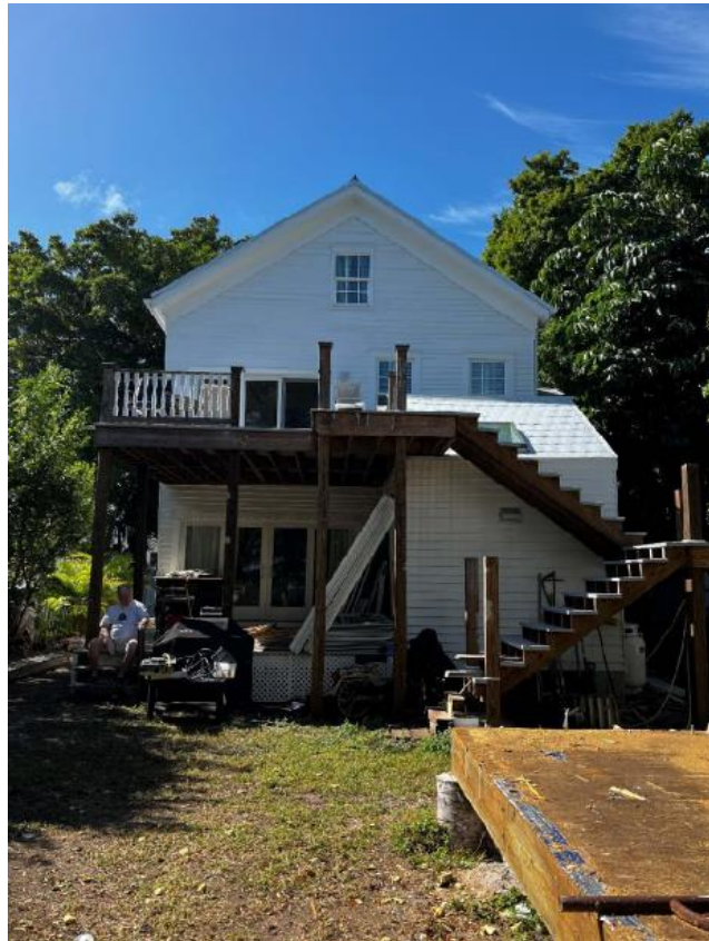
Photo of rear of house.
