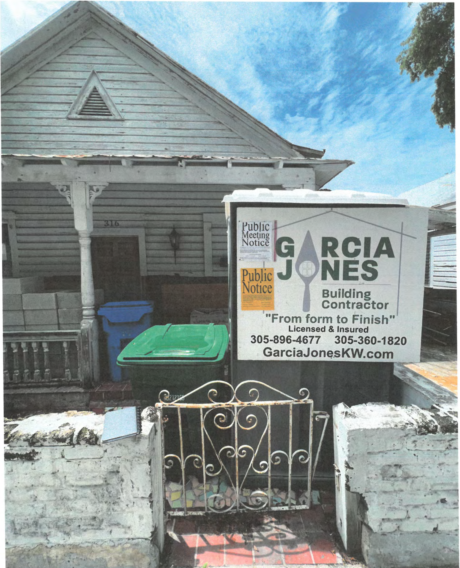
316 SOUTHARD ST. - HARC POSTING - 2
