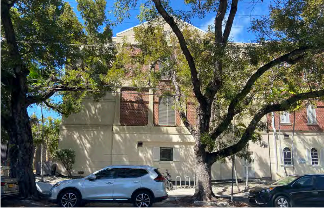
530 White Head Street [across the street]- Lester Building, Monroe County Offices
