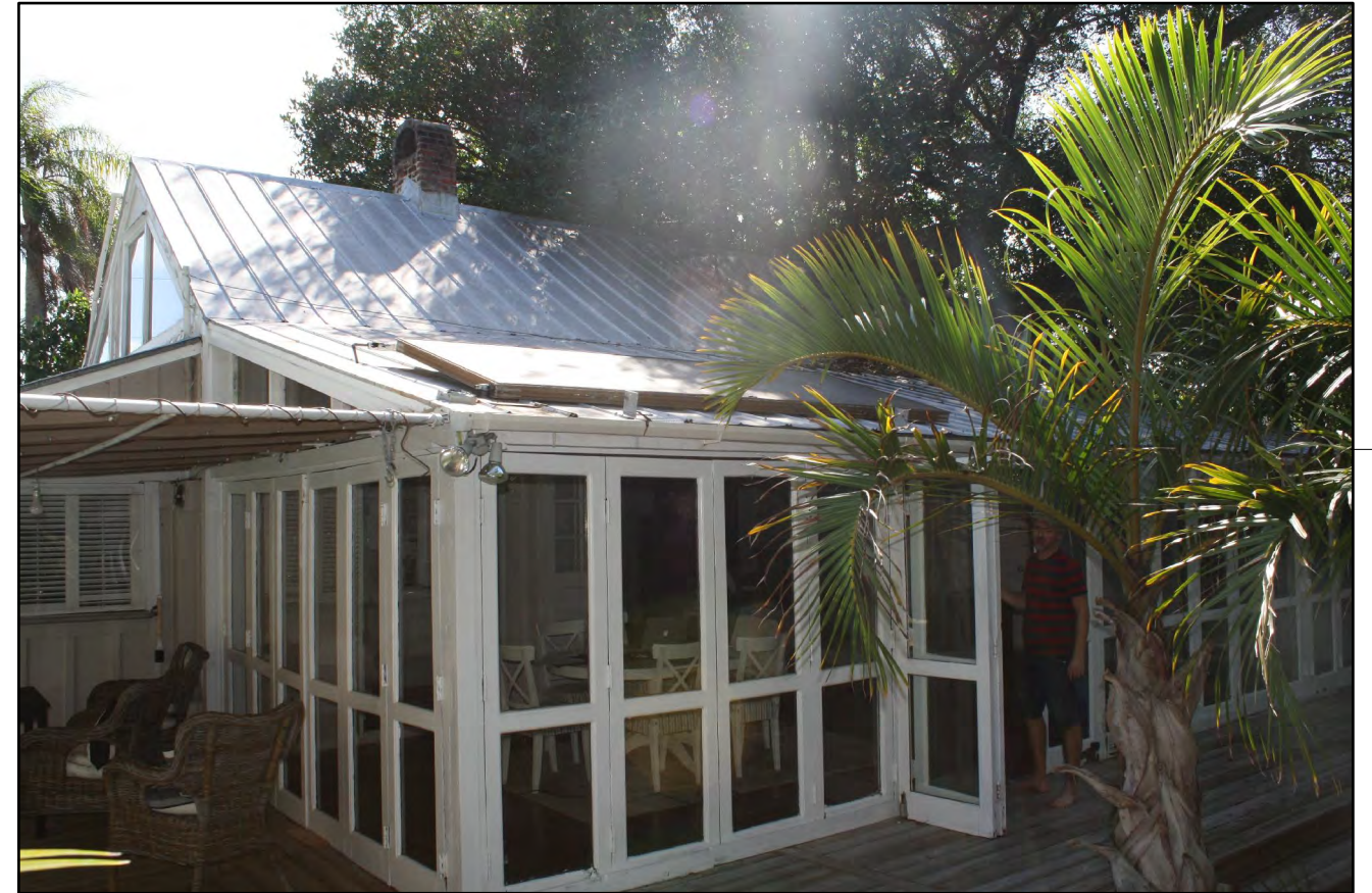
PHOTOGRAPH OF THE ADDITION TO THE NORTH OF THE HISTORIC STRUCTURE FROM THE SIDE YARD
