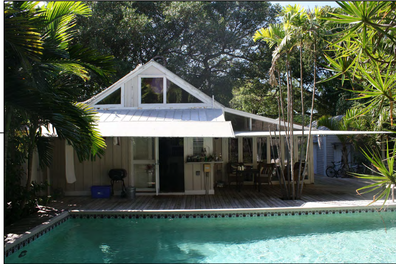
PHOTOGRAPH OF THE MAIN STRUCTURE FROM REAR YARD
