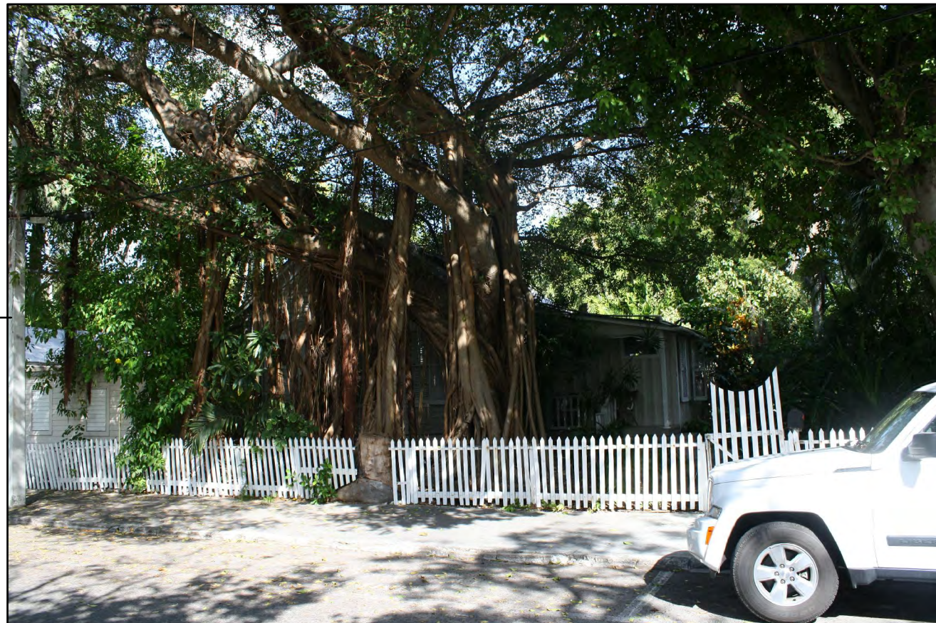
PHOTOGRAPH LOOKING AT THE ADDITION TO THE SOUTH OF THE HISTORIC STRUCTURE FROM MARGARET STREET
