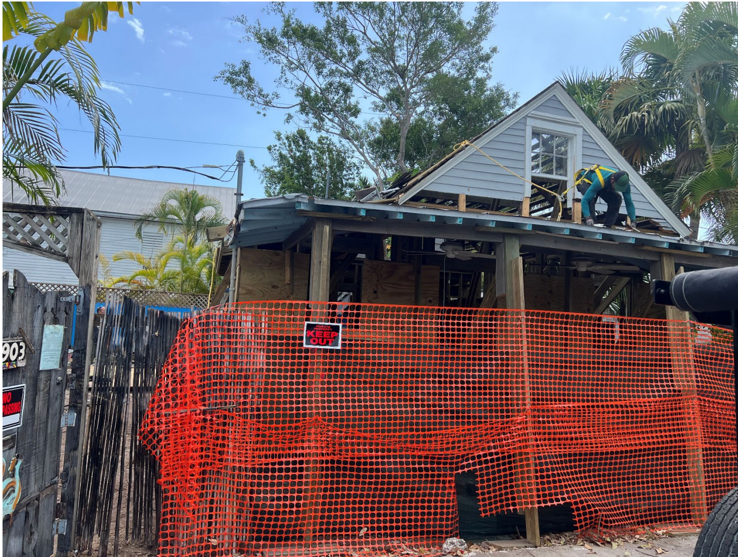
2. Existing Structure View – from Frances St.
