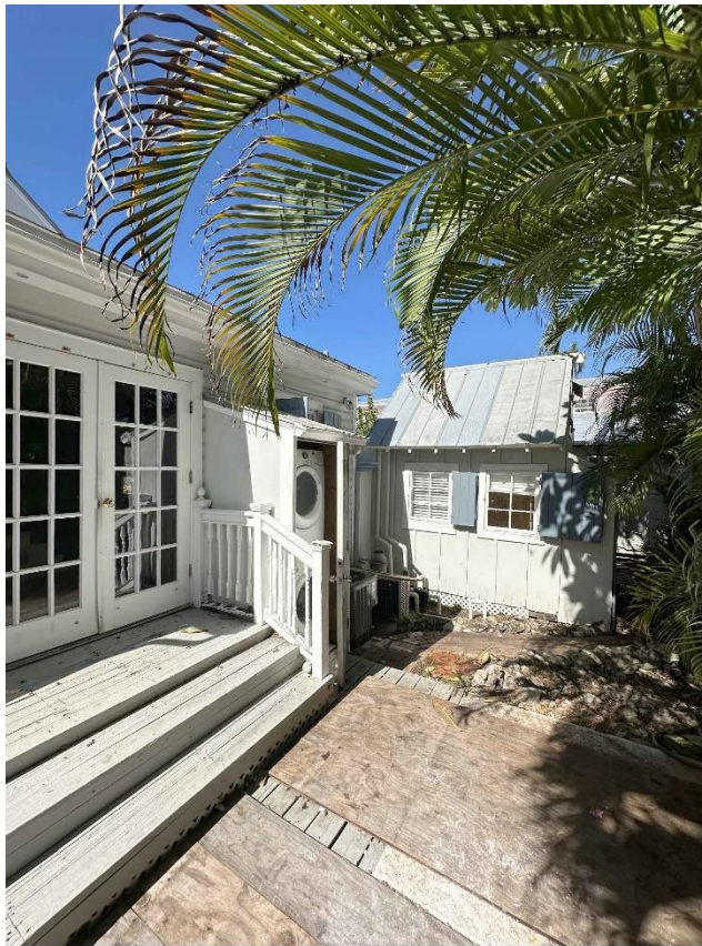
Partial Rear Elevation with Accessory Structure.
