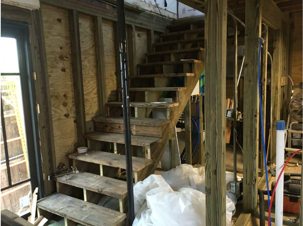
904 Olivia interior stairs (in progress renovation)
