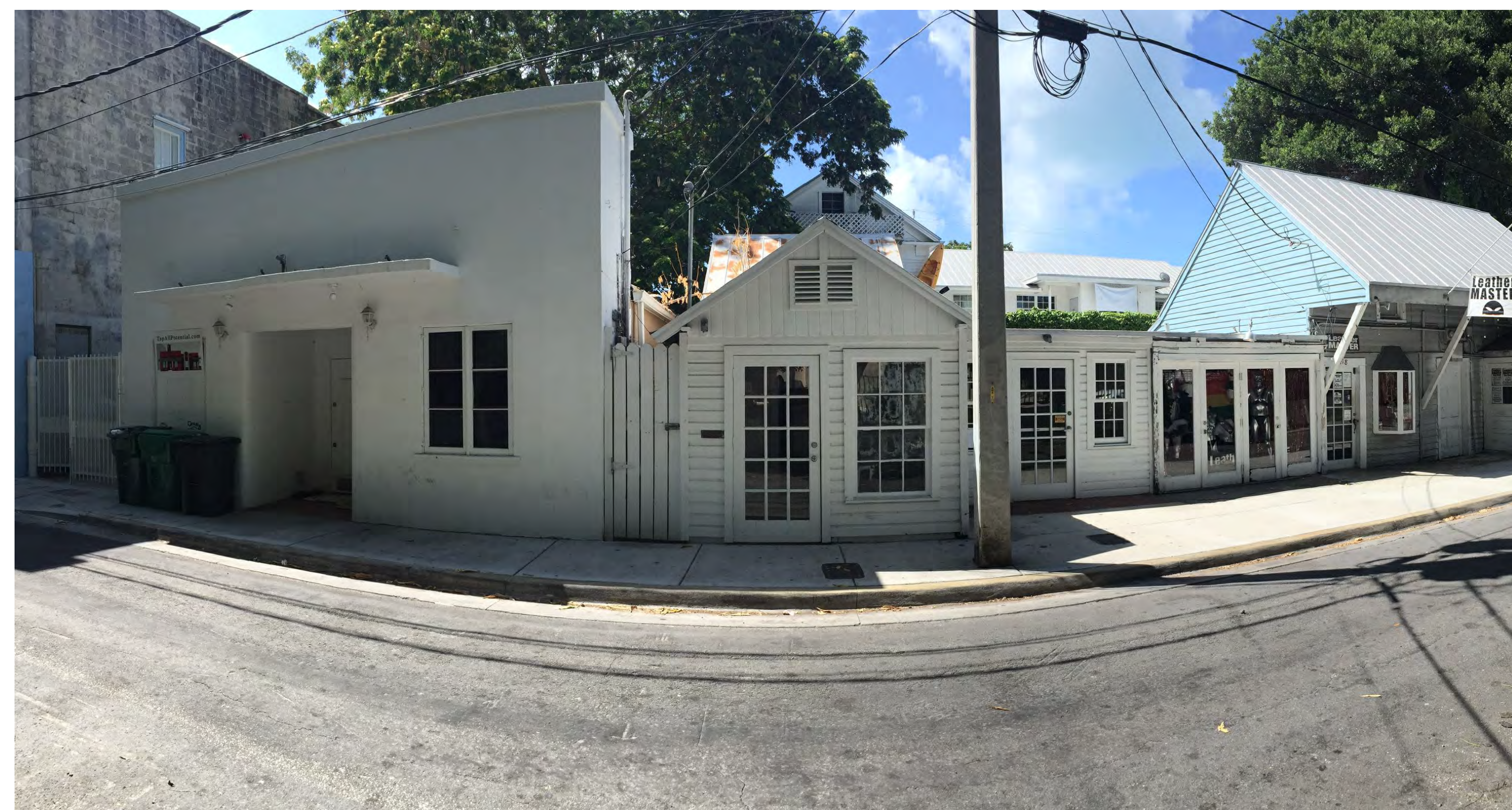
3 PHOTOGRAPH OF STREET ELEVATION (EXISTING WEST ELEV.) SCALE: N.T.S.
