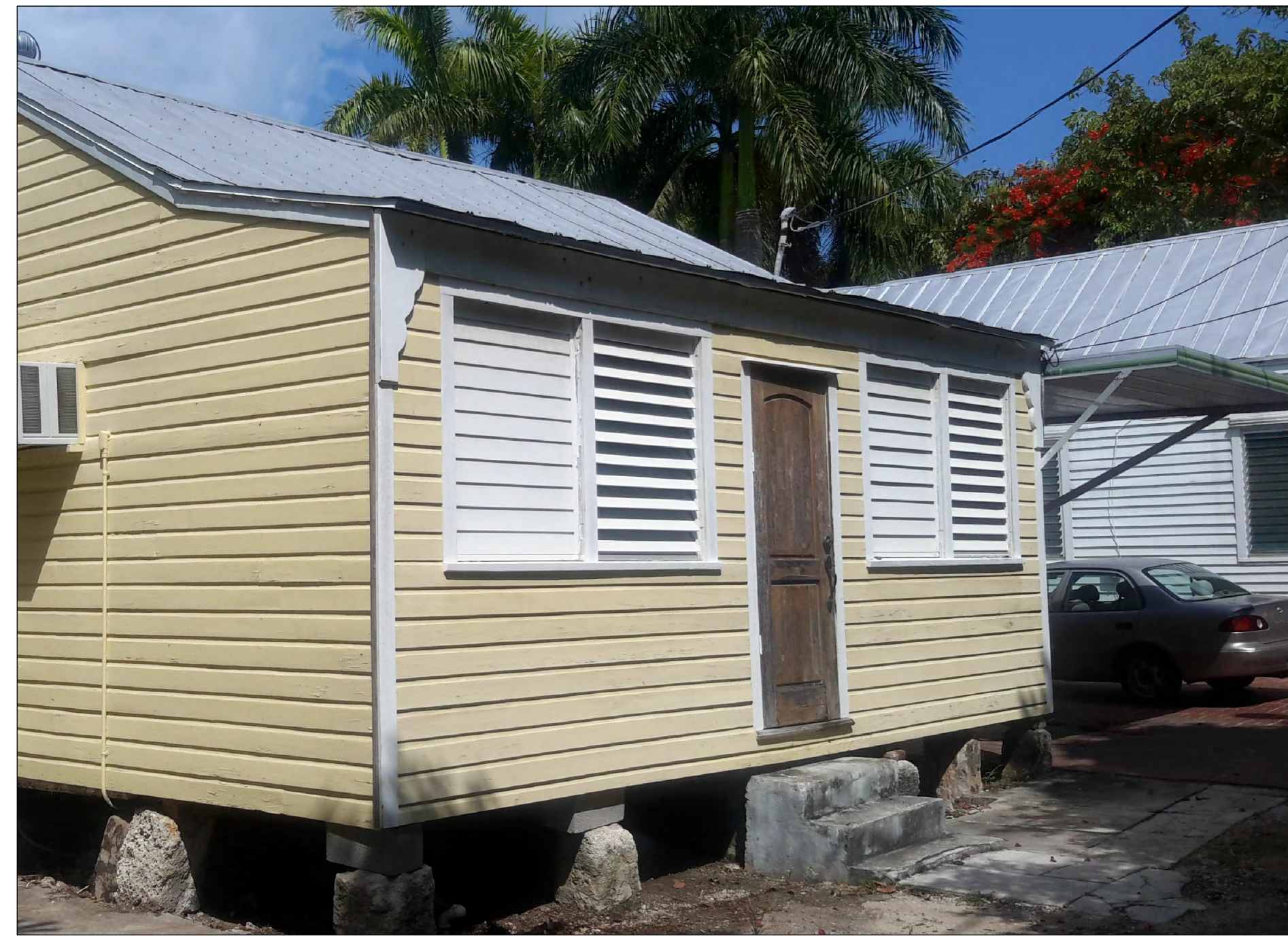
STREET VIEW (EXISTING) (VIEW FROM KNOWLES LANE)
