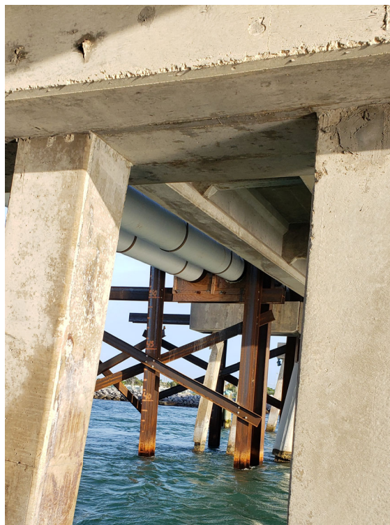
Figures 2. Side view of temporary stabilization.
