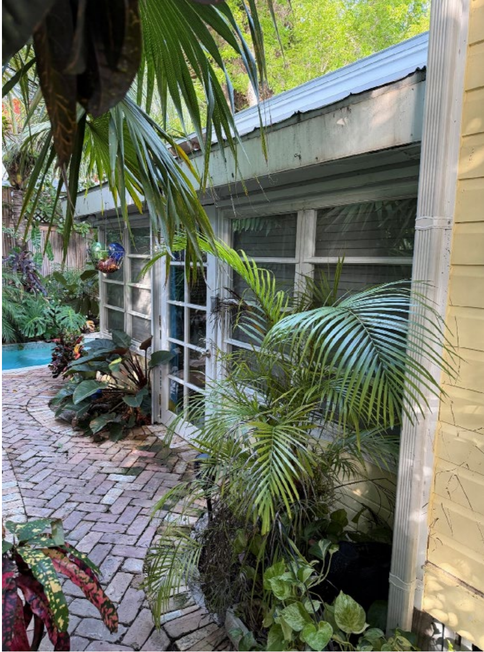
Photo of Rear of Property Under Review Showing Addition Proposed to be Demolished.
