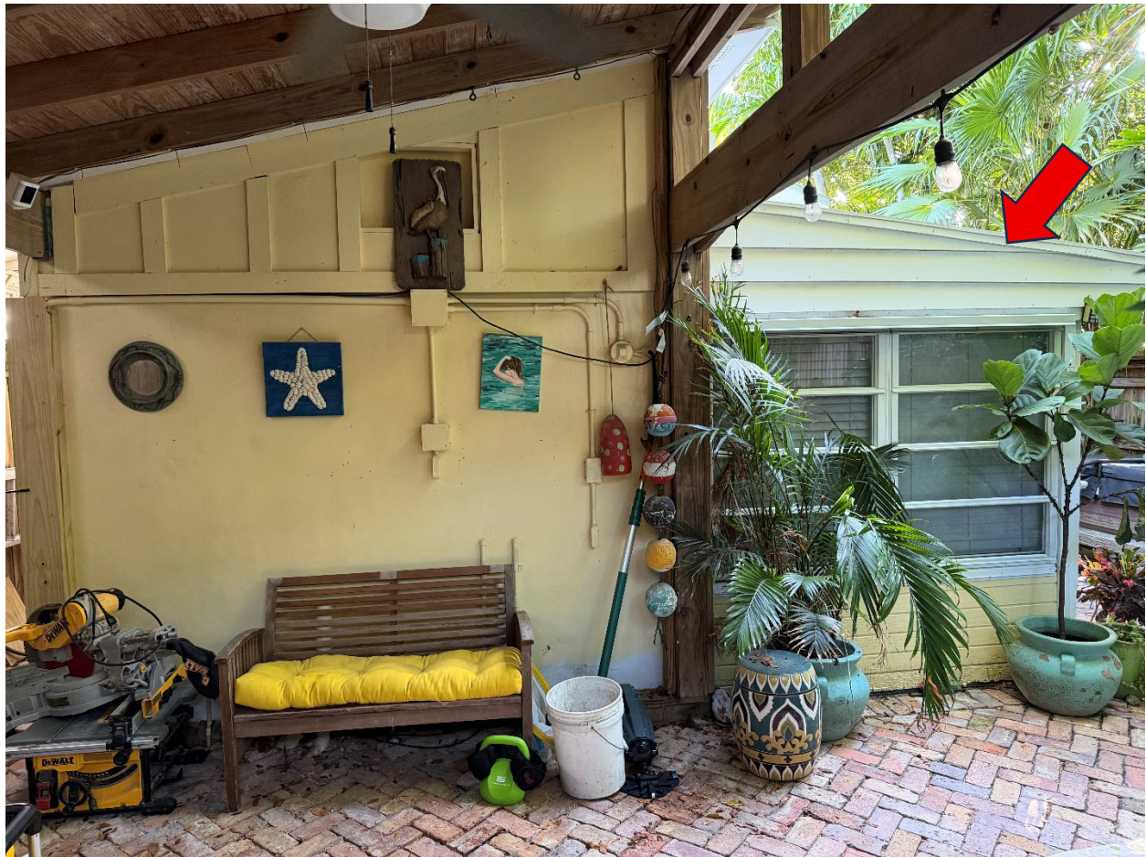
Figure 5 – Rear view, beneath open porch. Structure to be demolished indicated by red arrow.
