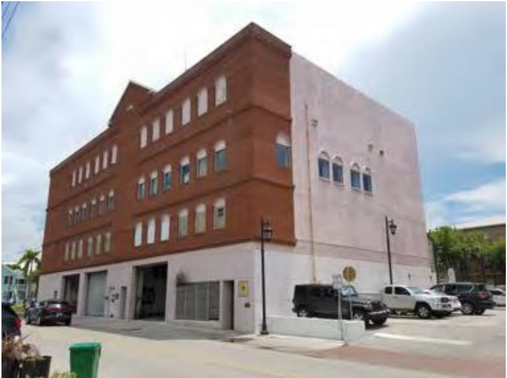
521 Thomas Street, Key west, Florida 33040 SITE VISIT
