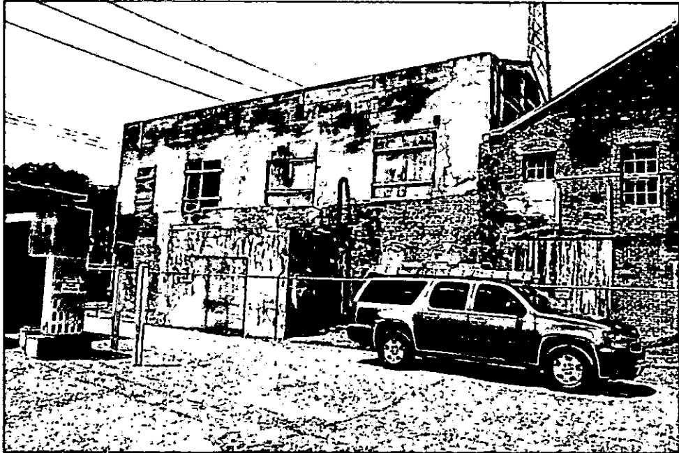
PHOTOGRAPH 5 (BUILDING IV AND V)
