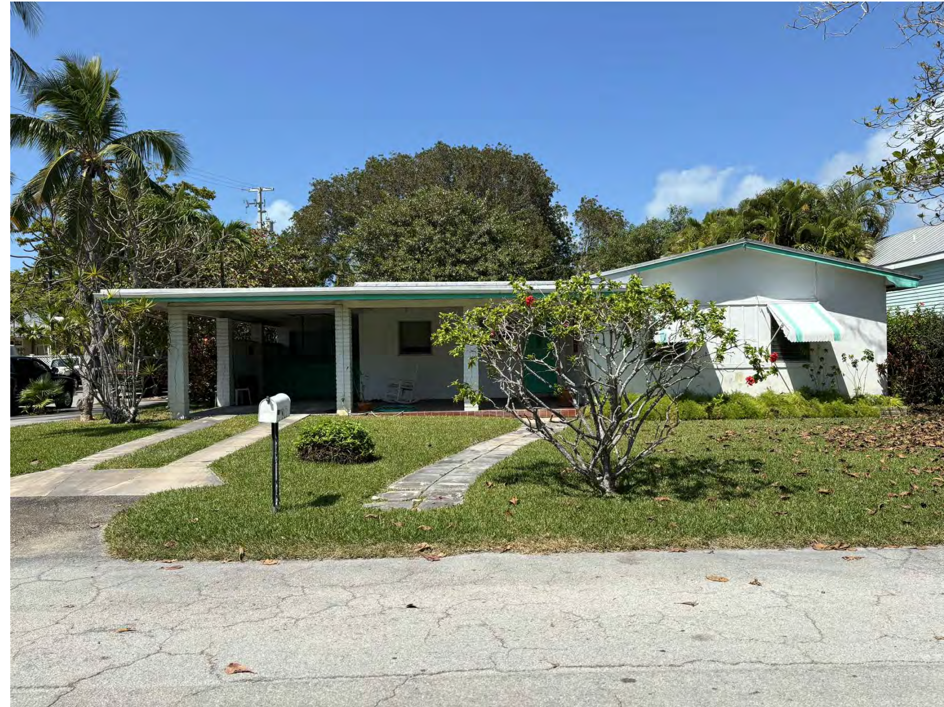
4 A8 VIEW OF THE FRONT OF THE HOUSE (EXISTING SOUTH ELEVATION) SCALE: N.T.S.
