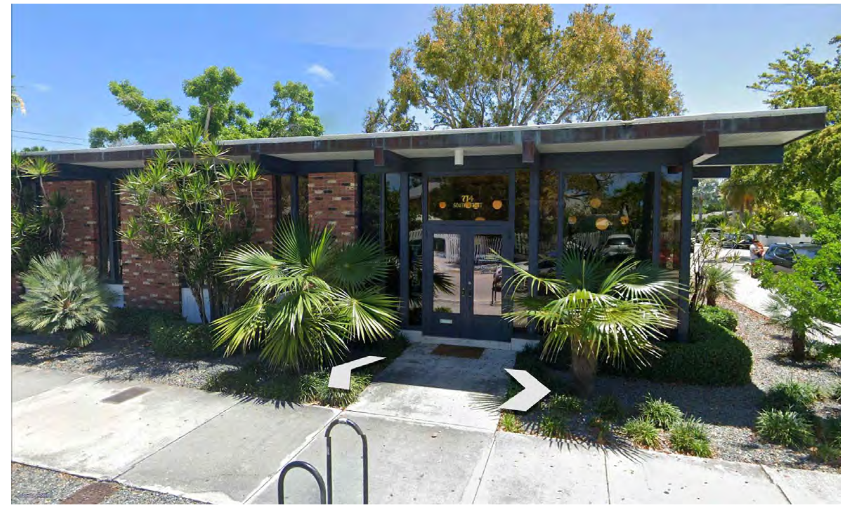
8 714 SOUTH ST. (ADJACENT PROPERTY TO NORTH) A7 SCALE: N.T.S.
