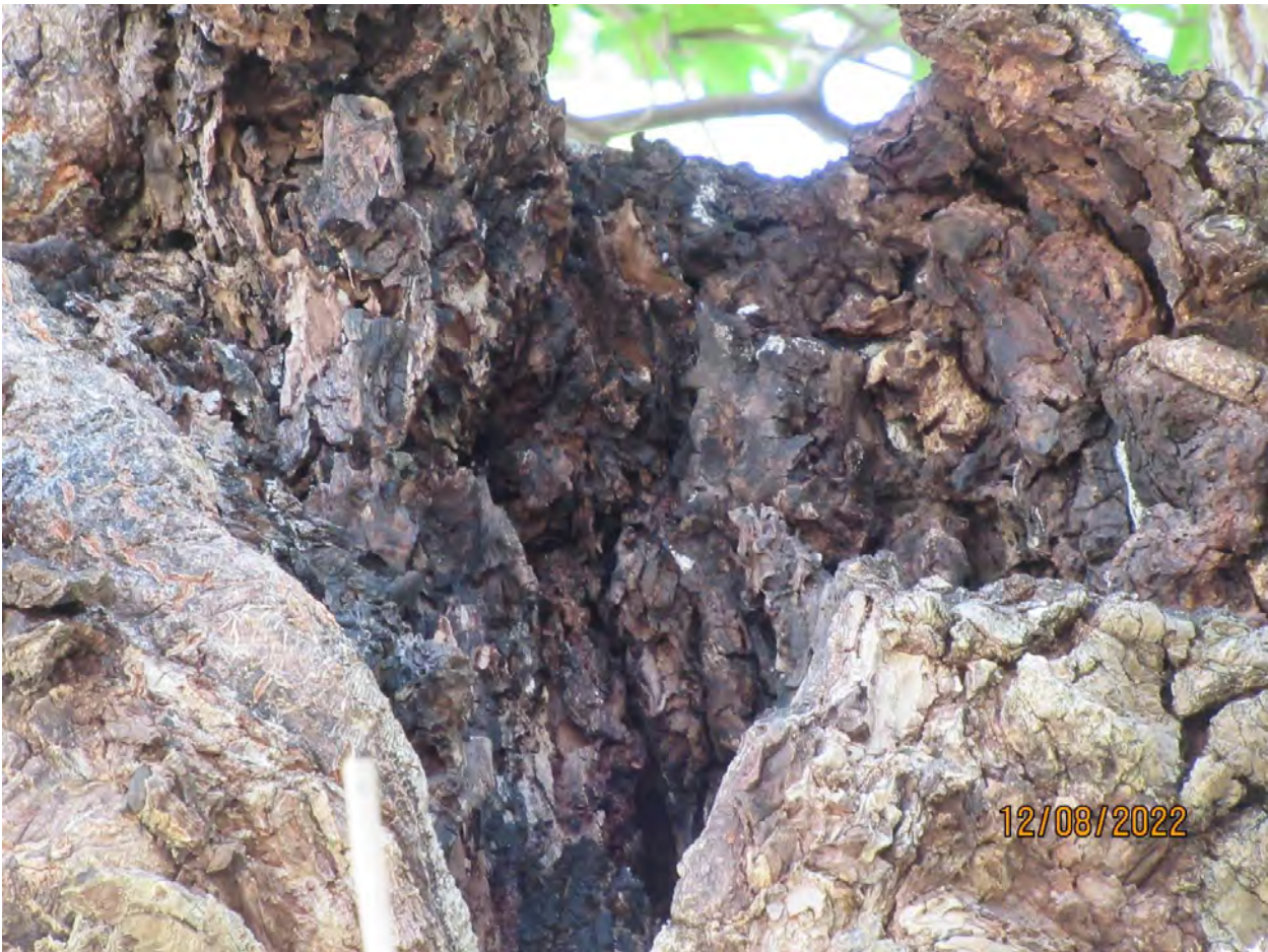
Close up view of old decay area, view 2.
