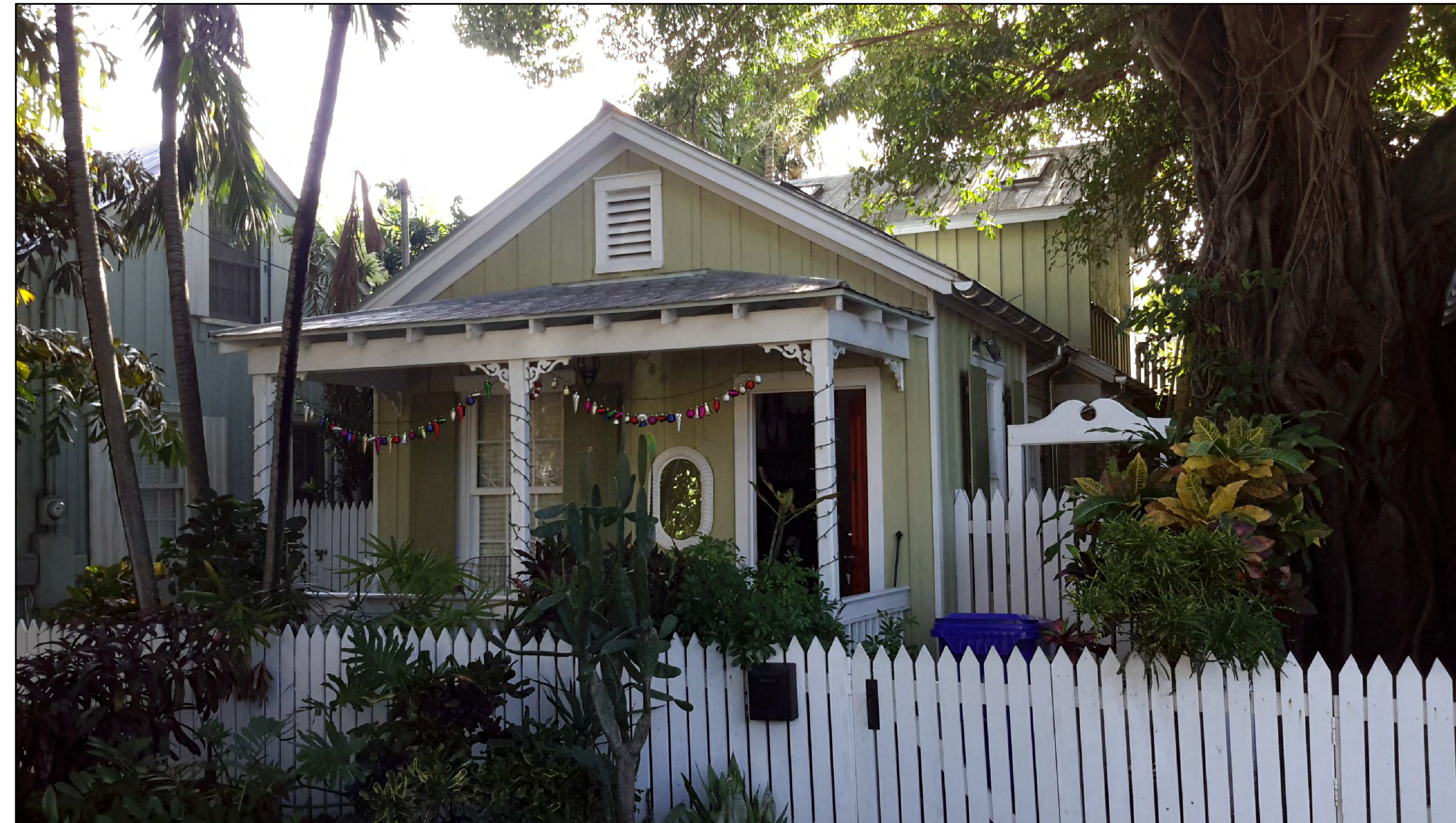
VIEW FROM CARSTON LN.
