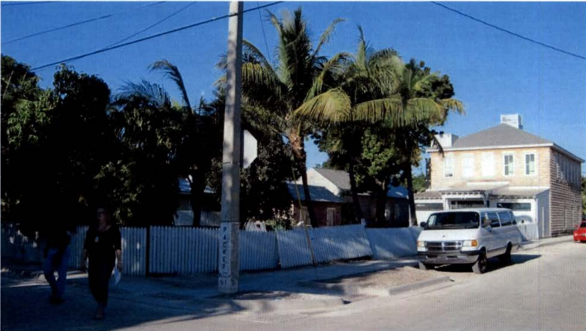
8. Northeast corner of Packer Street: One potential planting area, we would like to transplant (1) Christmas Palm.
