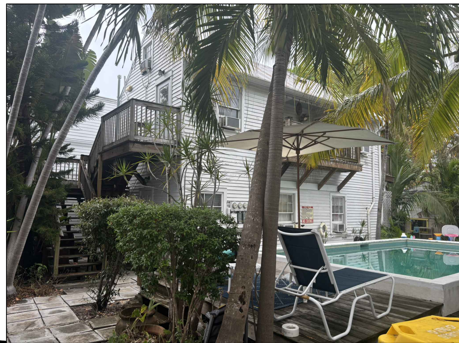
1 ADJACENT TWO STORY BUILDING VIEW FROM YARD PI SCALE: N.T.S
