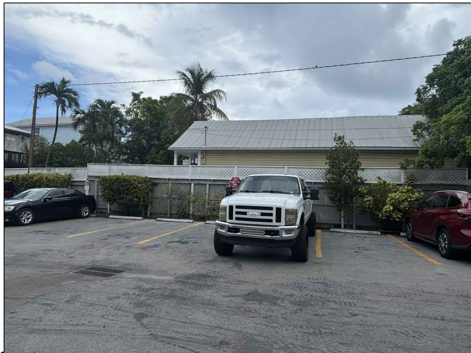
5 716 DUVAL ST ONE AND A HALF STORY BUILDING VIEW FROM PARKING LOT OFF OF SAMARITAN LN PI SCALE: N.T.S
